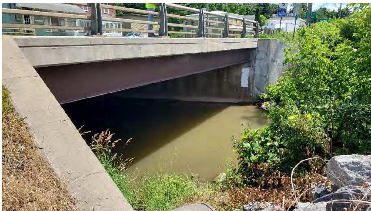
Figure 7-38. NY-5/Genesee Street bridge, Oneida, NY.
