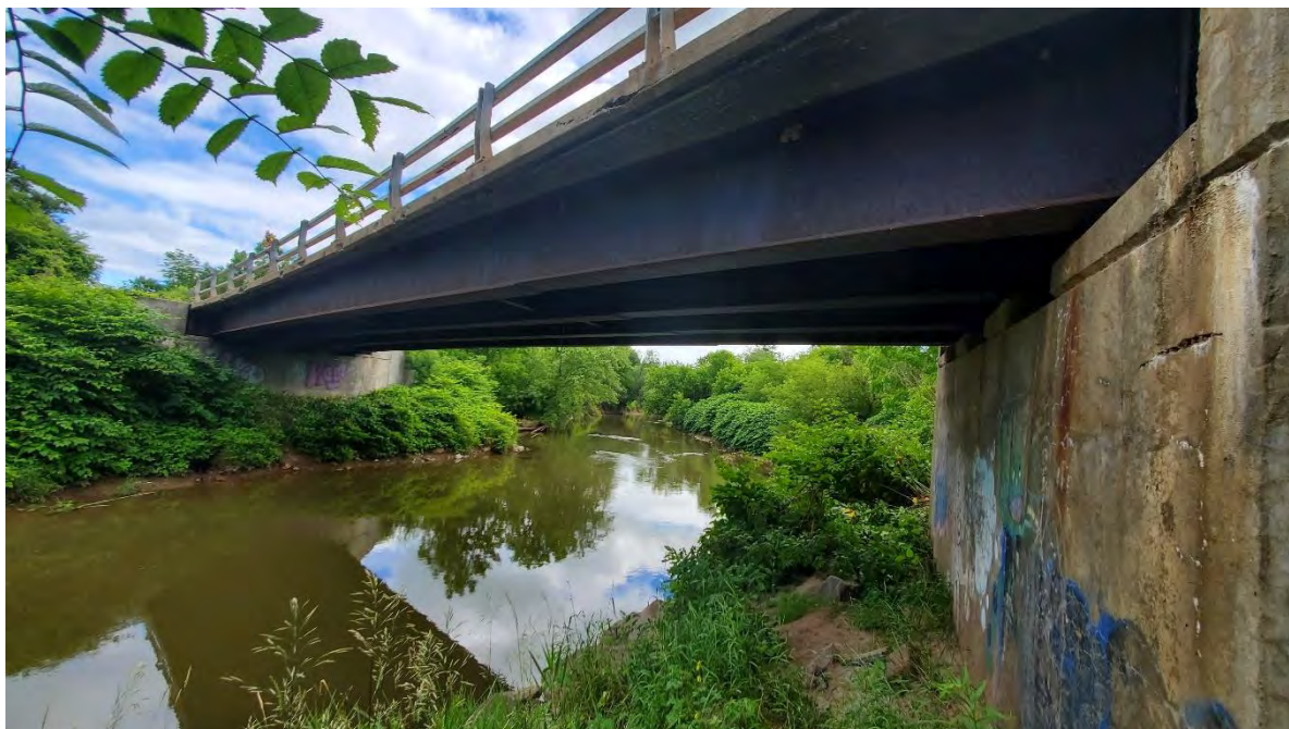
Figure 7-14. Bennett Road bridge, Oneida, NY.
