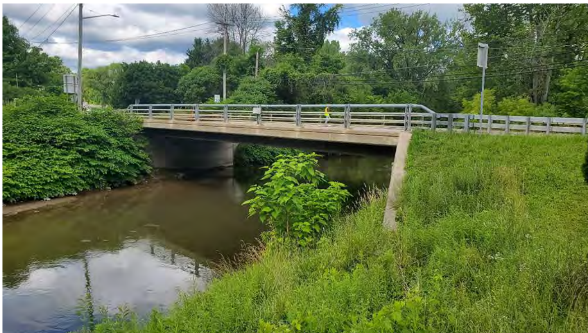
Figure 7-22. Sconondoa Road bridge, Oneida, NY.
