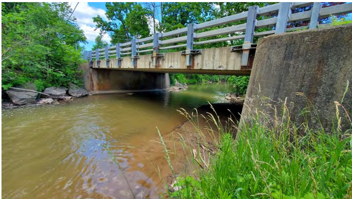
Figure 7-63. CR-51 Kenwood Avenue/CR-25 Hamilton Street bridge, Oneida, NY.
