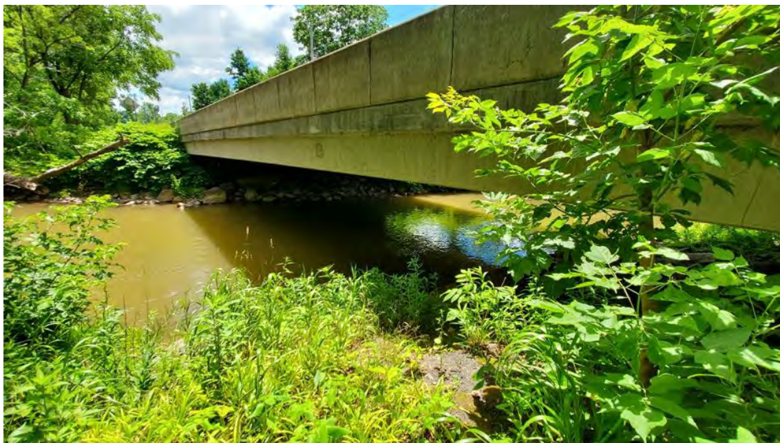
Figure 7-50. Middle Road bridge, Oneida Castle, NY.
