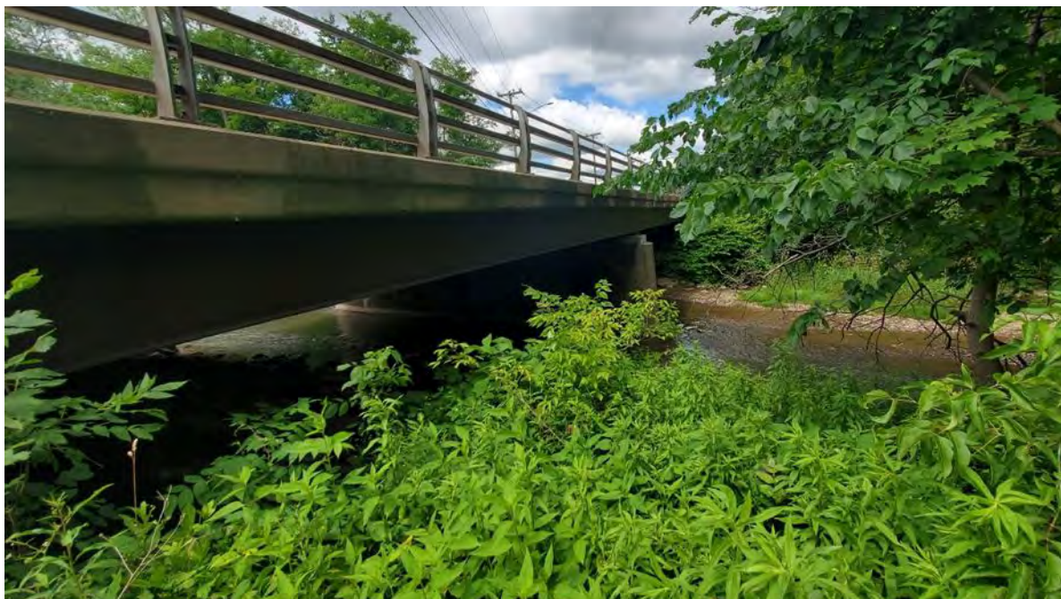
Figure 7-25. Prospect Street bridge, Oneida, NY.
