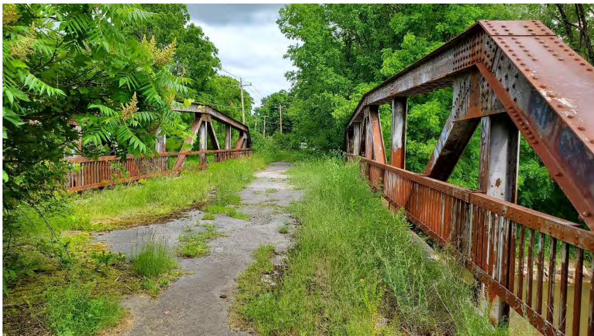
Figure 7-9. Old State Route 46/Oneida Street bridge, Oneida, NY.
