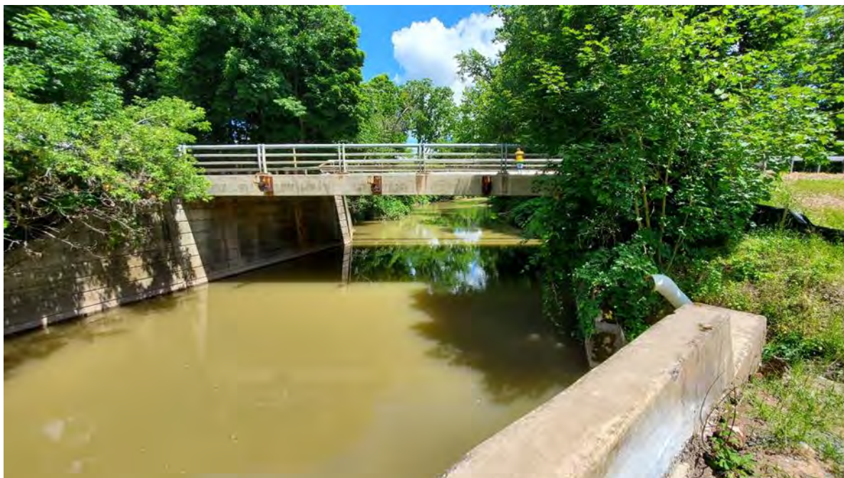
Figure 7-58. Sherrill Road/CR-51 Kenwood Avenue bridge, Sherrill, NY.
