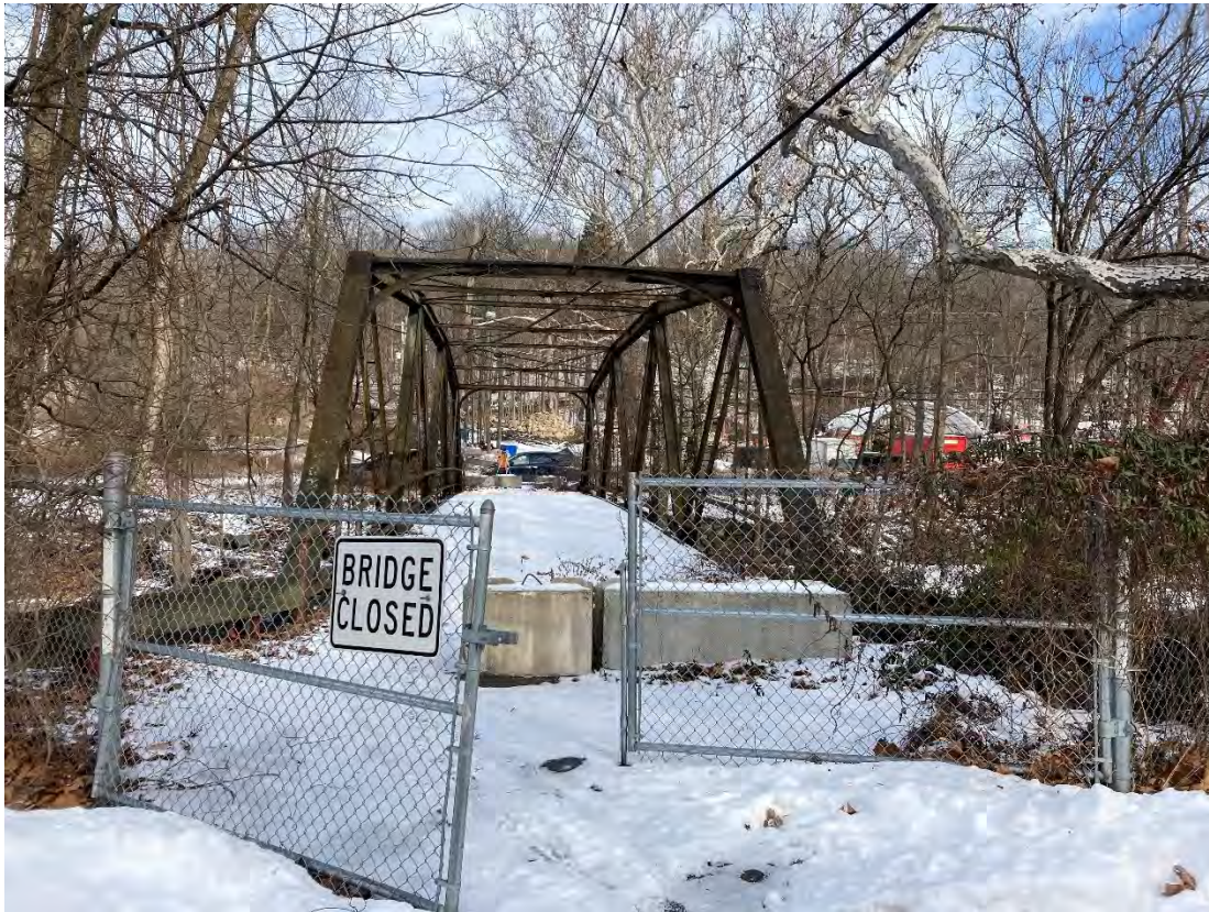
Figure 4-17: Out of service but pedestrian-accessible Bridge Street bridge at STA 138+00
