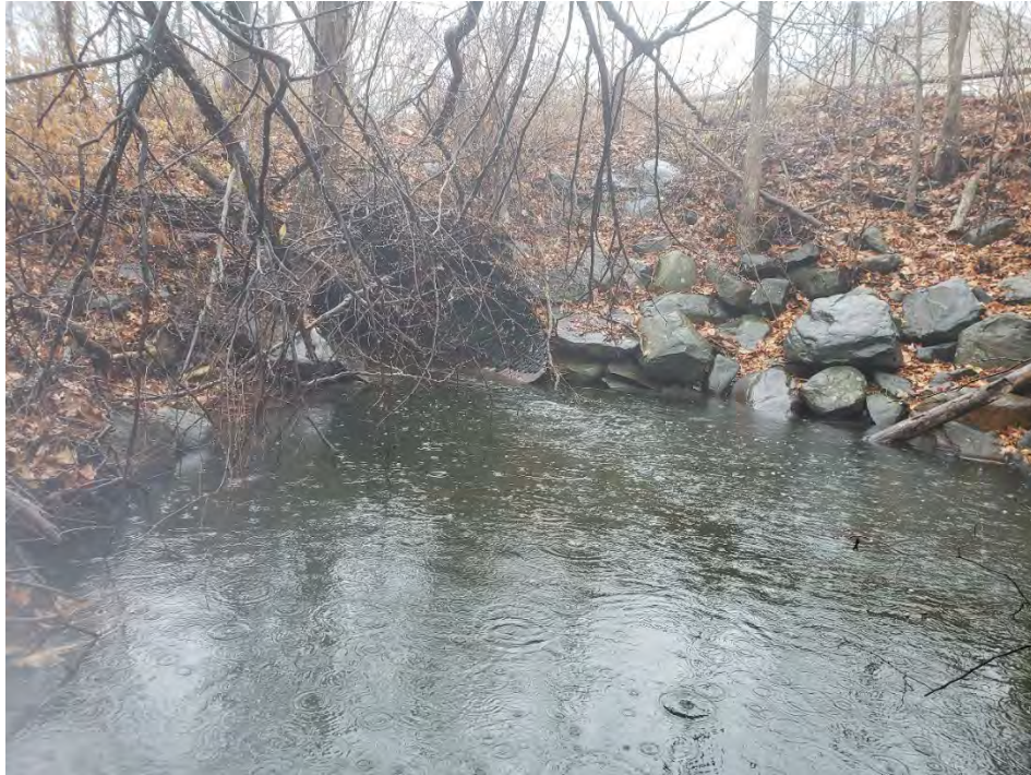
Figure 4-60: Downstream outlet of Brookside Drive East culvert crossing
