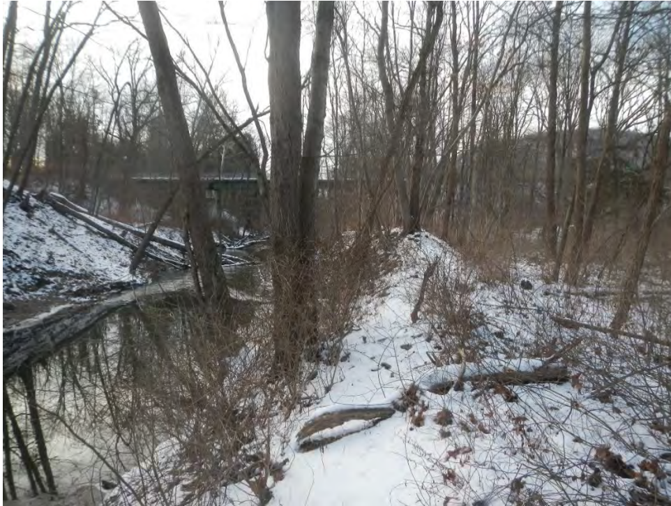
Figure 4-33: Looking downstream towards Kanawauke Road bridge, visible through the trees in the upper-left quadrant of the image. Centered in the image is an approximately 6-foot-tall right bank berm.
