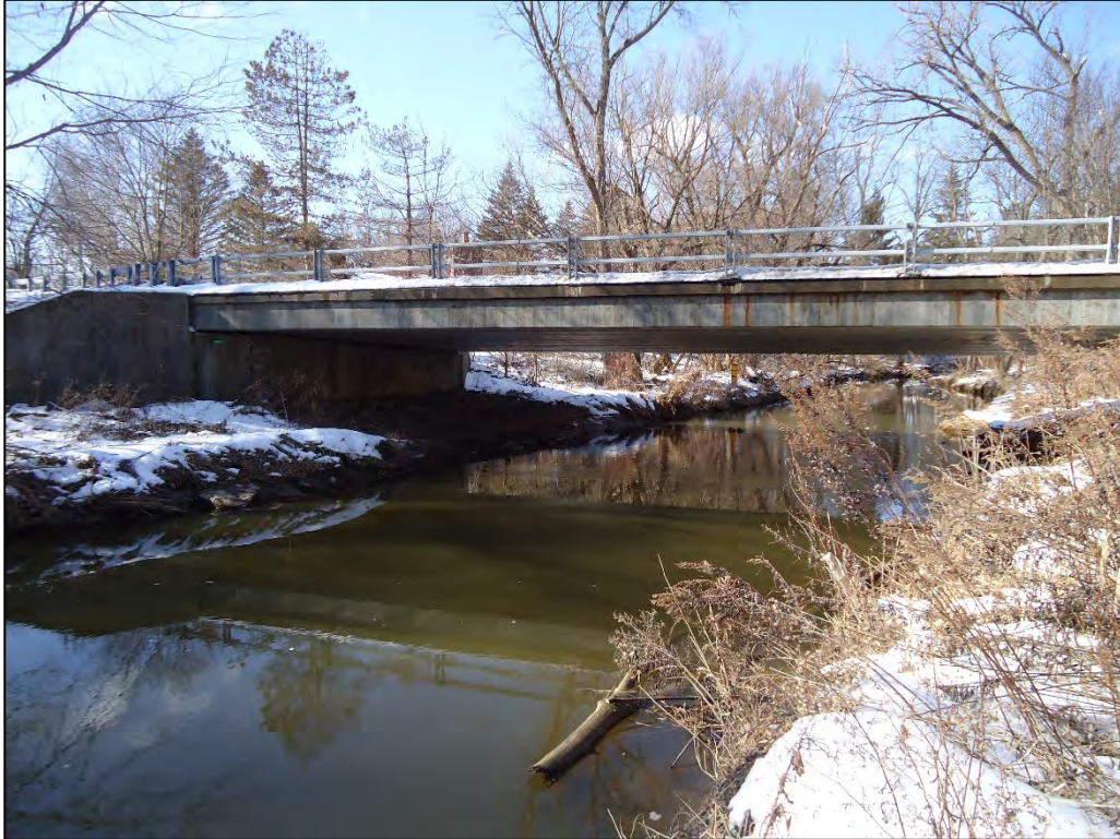
Photo D-3. Upstream face of Hopkins Road Bridge over Ransom Creek (2/17/2020)
