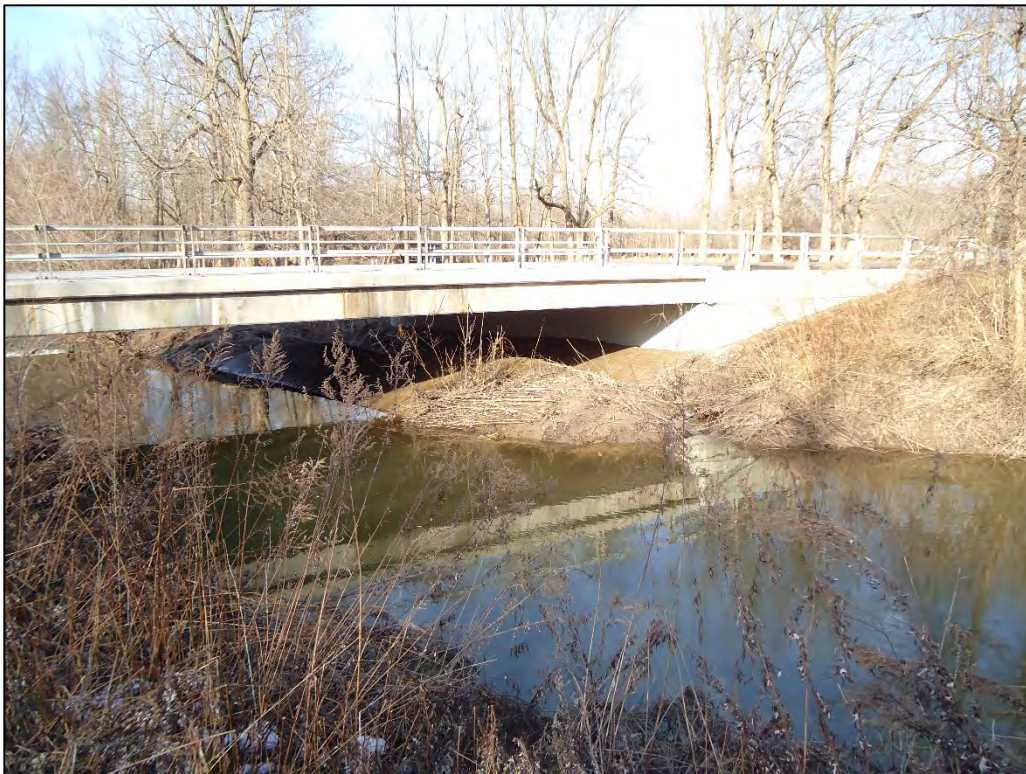
Photo D-7. Upstream face of Dodge Road bridge crossing Ransom Creek (3/5/2020)
