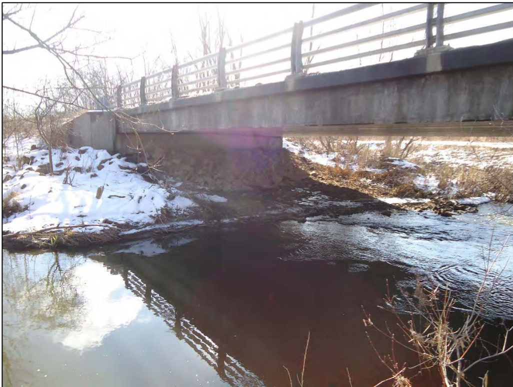
Photo D-5. Upstream face of New Road bridge over Ransom Creek (2/17/2020)
