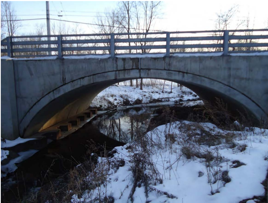
Photo 3. Downstream Face of Miles Road Bridge over Ransom Creek
