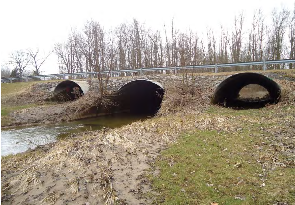
Photo 2. Downstream Face of Glen Oaks Drive Culverts over Ransom Creek
