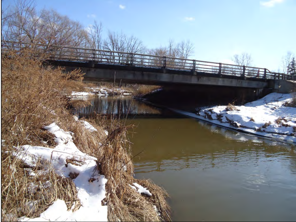
Photo D-4. Downstream face of Millersport Highway bridge over Ransom Creek (2/17/2020)
