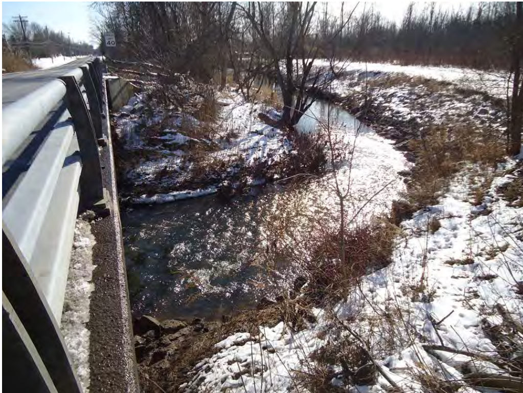
Photo 1. Severe Bend in Ransom Creek Downstream of New Road Bridge
