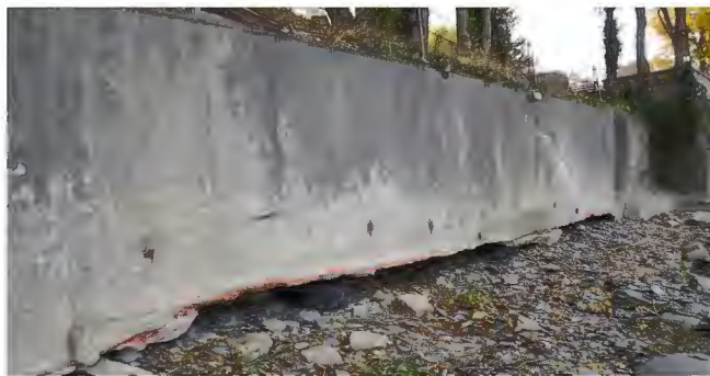
PHOTO 17. Undermining of a seawall along Lake Erie
