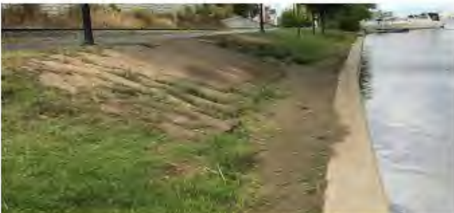
PHOTO 18. Bulkhead on the west side of the Genesee River that was damaged by overtopping. Recently repaired by backfilling with soil, and planted. Photo taken in 2019 after the high water level events.
