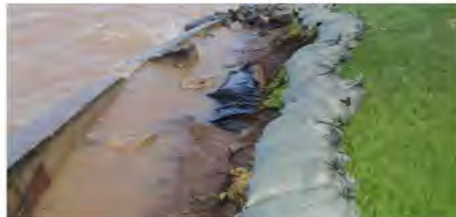
PHOTO 19. Wall that was damaged by overtopping and undermining, Lyndonville, N.Y.
