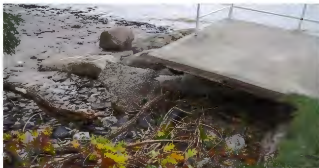
PHOTO 16. Flanking observed at a bulkhead located on Lake Erie
