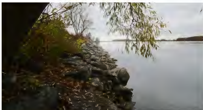
PHOTO 8. Stone revetment with a vegetative buffer in Waddington, N.Y.
