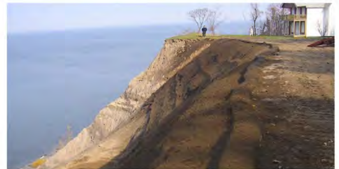
PHOTO 12. Placement of erosion control and a seed mix on a re-graded slope on Lake Ontario near Sodus Bay. Construction was completed in 2008.
