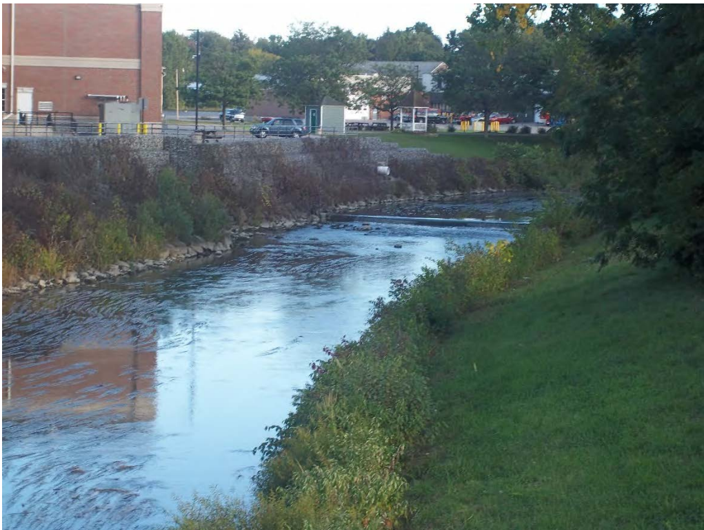
Photo D-4. Small dam upstream from pedestrian bridge at Walnut Street
