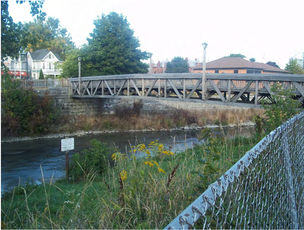
Photo D-1. Downstream face of pedestrian bridge at Walnut Street
