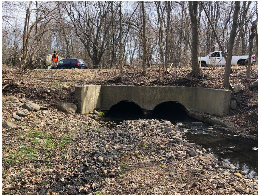
Figure 4-29: Looking downstream at the inlet of East Blossom Road culverts
