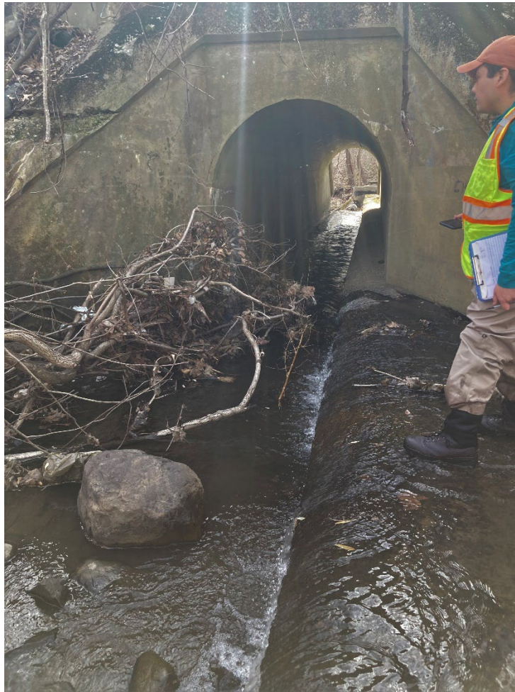
Figure 4-34: Looking downstream at the inlet of the Conrail bridge structure
