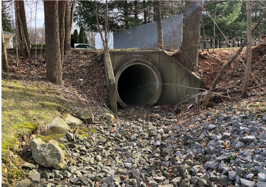
Figure 4-41: Looking downstream at the inlet of the Olympia Lane culvert
