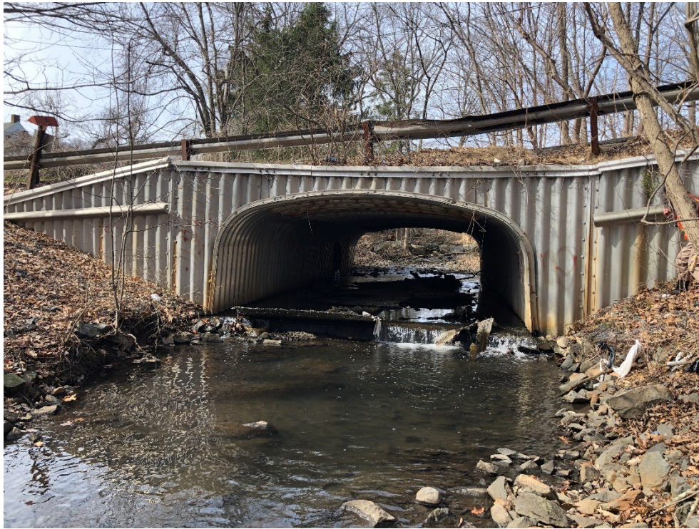
Figure 4-23: Looking upstream at the outlet of Christmas Hill Road culvert
