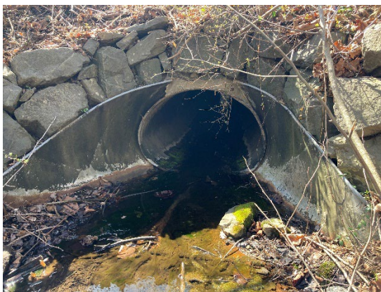
Figure 4-10: Relief culvert along Hillside Avenue: Single inlet (L) splits into two outlet pipes (R)
