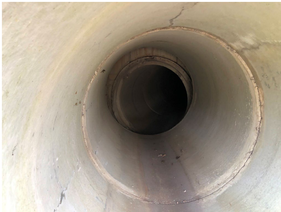
Figure 4-42: Looking downstream inside the Olympia Lane culvert at the 30-degree bend
