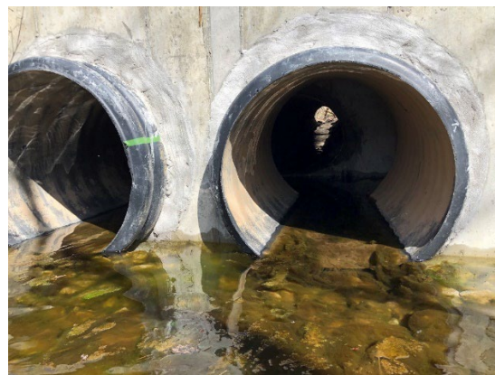
Figure 4-10: Relief culvert along Hillside Avenue: Single inlet (L) splits into two outlet pipes (R)
