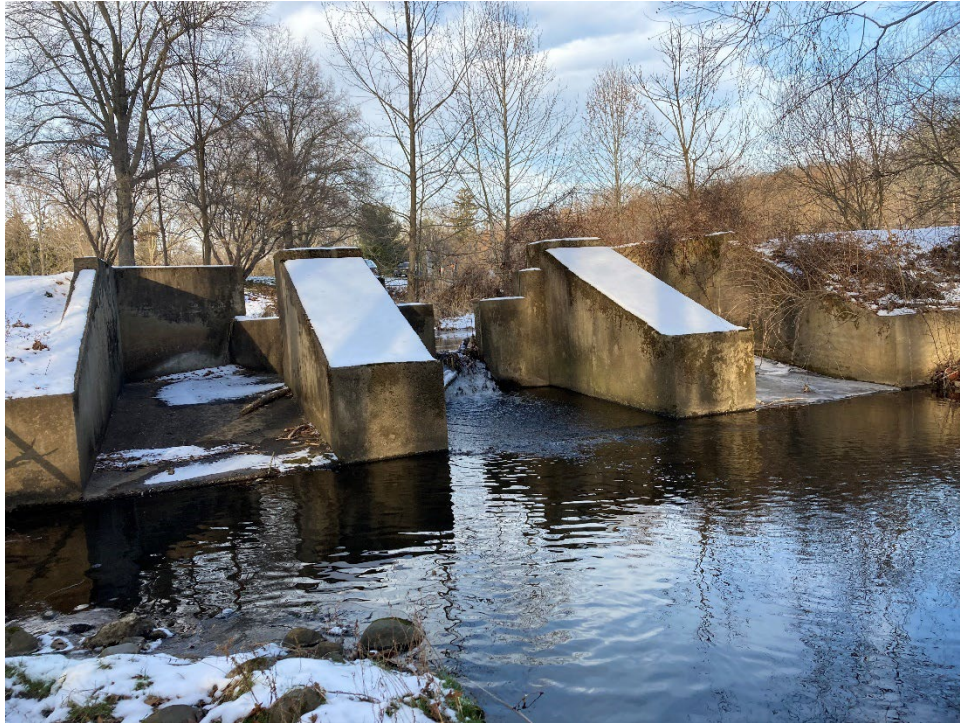
Figure 4-7: Outlet of dam downstream of Ascension Cemetery driveway
