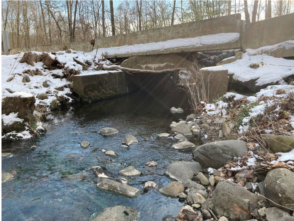
Figure 4-15: Inlet of South Monsey Road crossing of East Branch Saddle River
