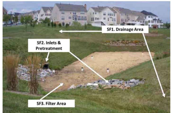
Figure 2.12.1. Key Areas for Level 1 Inspection of Sand and Organic Filters
