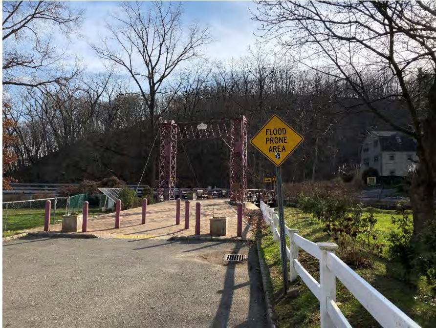
Figure 4-3 The historic Bridge Street bridge spans the Sparkill Creek as a pedestrian bridge just upstream of the Ferdon Avenue bridge.
