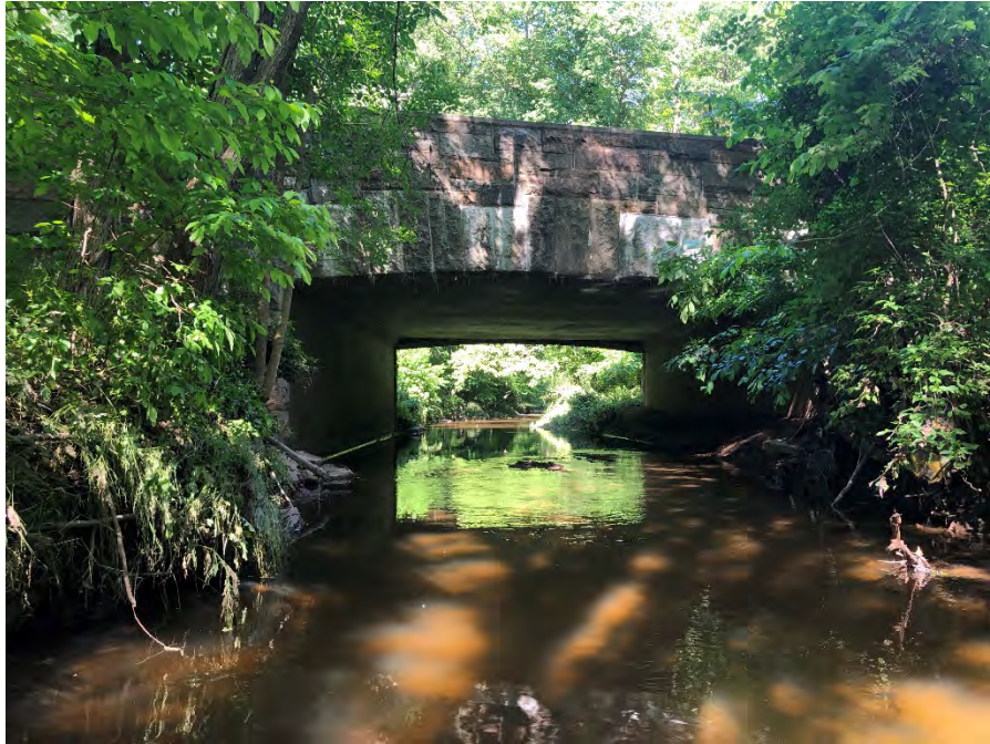
Figure 4-44: Looking Upstream at Northbound Palisades Interstate Parkway Bridge Outlet
