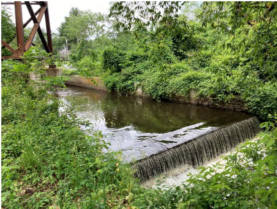
Figure 4-22: Boss Pond Dam Spillway
