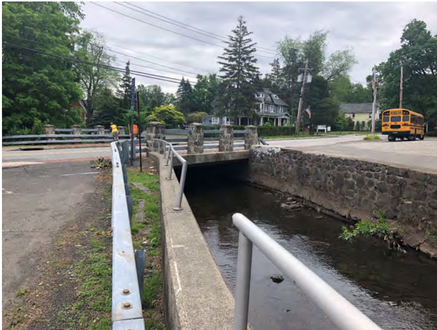
Figure 4-34: Washington Street Bridge and Channelized Section of Sparkill Creek
