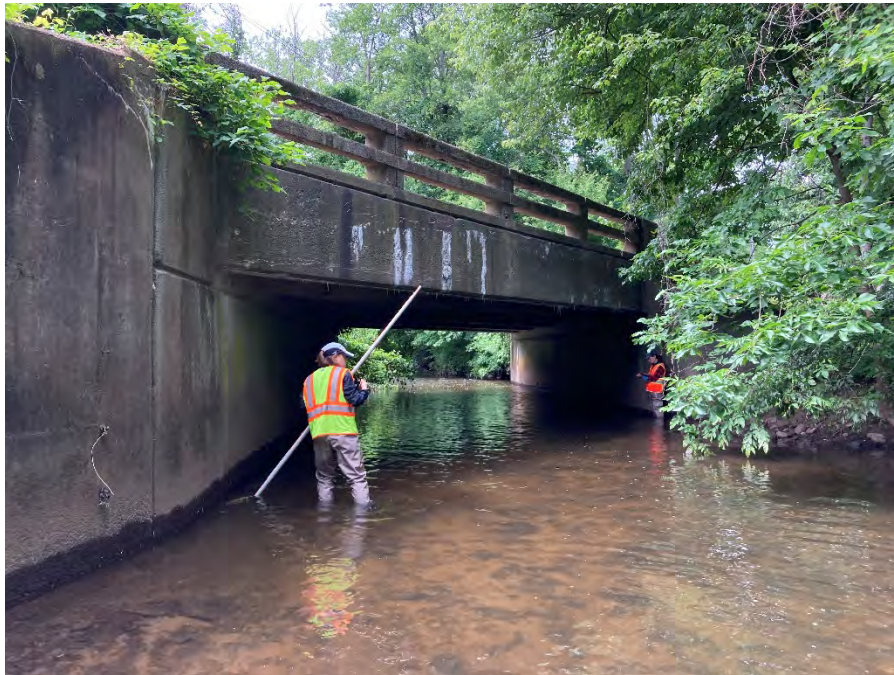
Figure 4-15: William Street Bridge
