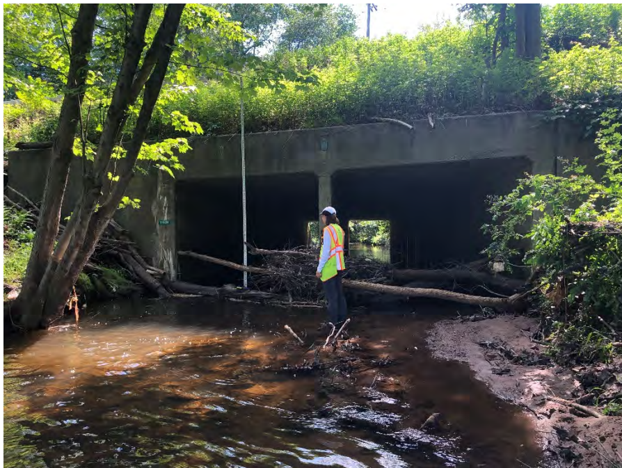
Figure 4-45: Looking Downstream at Route 303 Culvert Inlets
