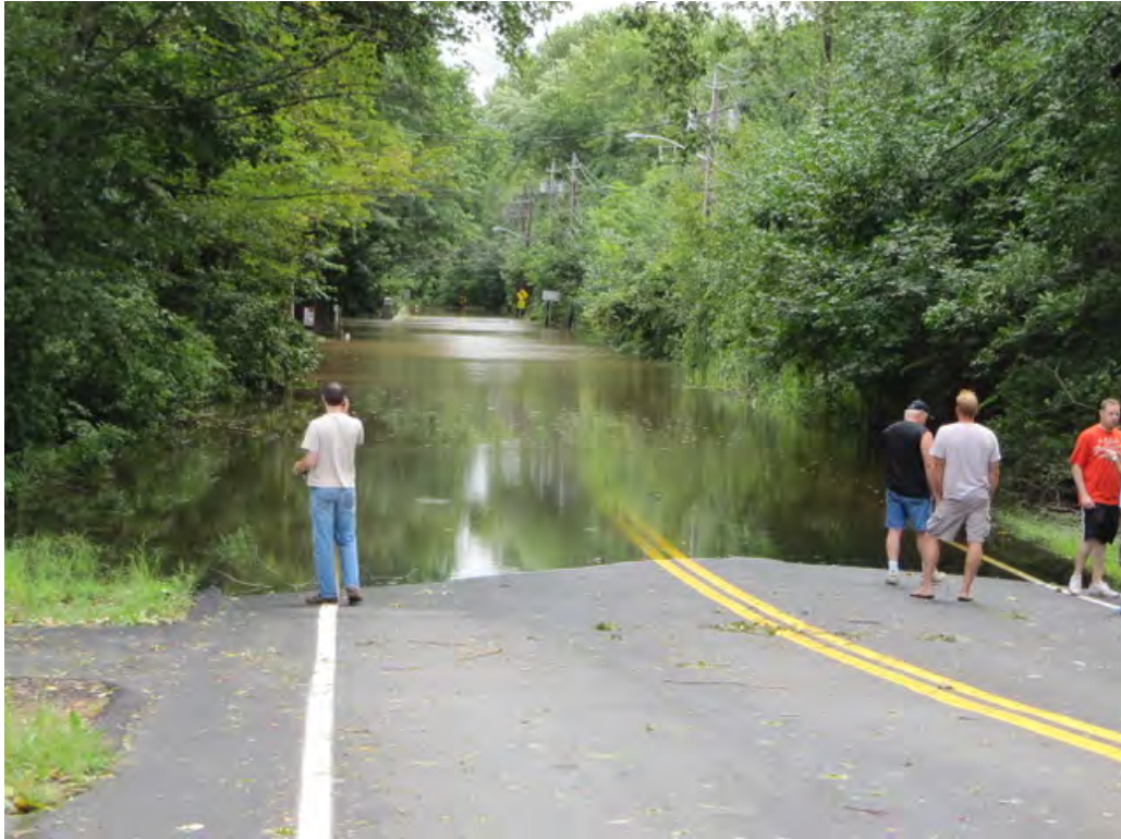
Figure 4-25: Oak Tree Road Bridge during Tropical Storm Irene (photo provided by Lawrence Vail)
