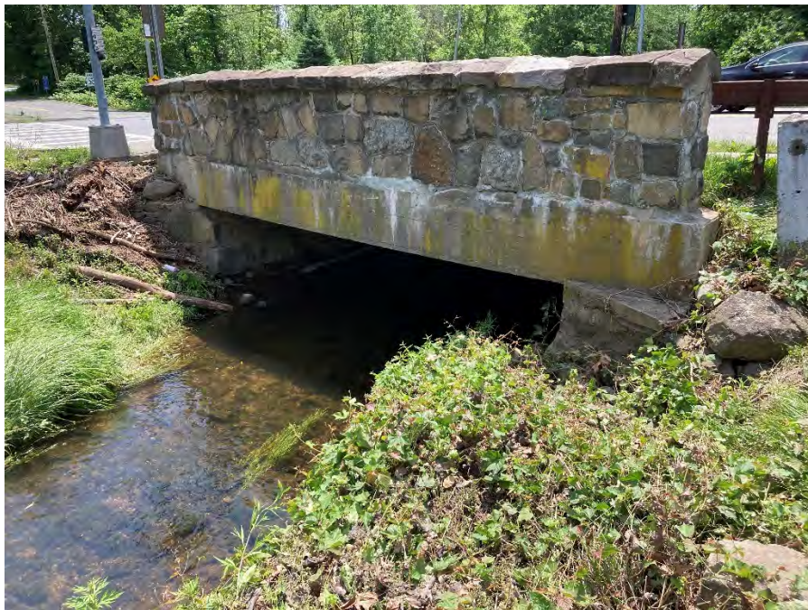
Figure 4-59: Looking Downstream at Mountain View Avenue Bridge Inlet
