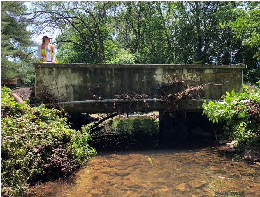
Figure 4-67: Looking Downstream at the Private Bridge to Innovative Plastics
