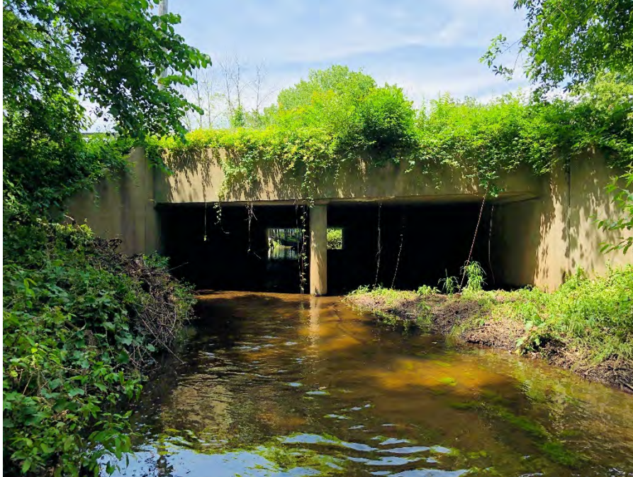
Figure 4-68 Looking Upstream at the Old School Lane/Orangeburg Road Culvert Outlets
