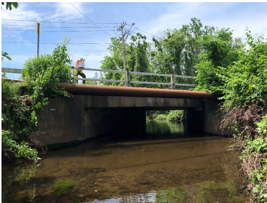
Figure 4-72: Looking Upstream at the Route 303 Bridge
