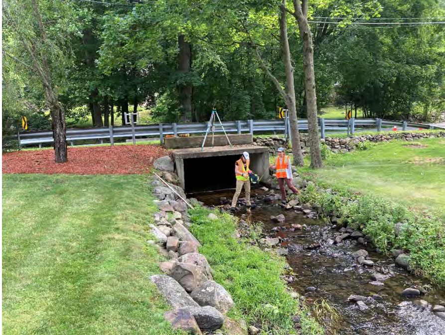
Figure 4-90: Looking Upstream at the Culvert that Carries Greenbush Road
