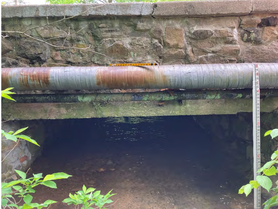
Figure 4-89: Looking Downstream at the South Greenbush Road Culvert Inlet
