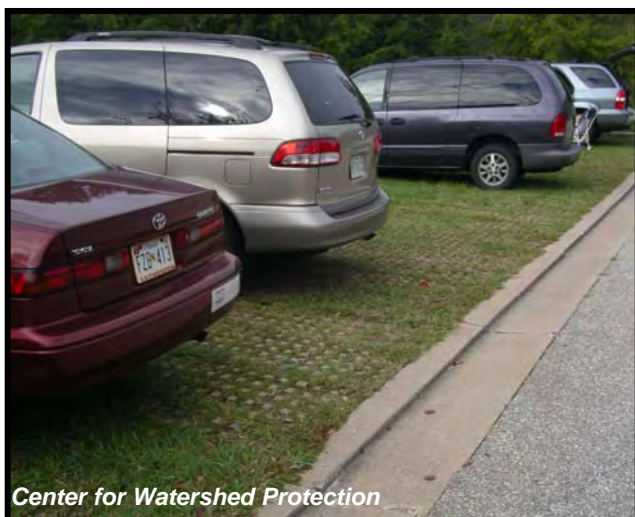
Figure 1: Application of Permeable Pavers
