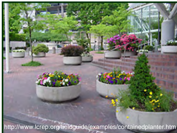
Figure 4: Contained stormwater planters made of concrete
