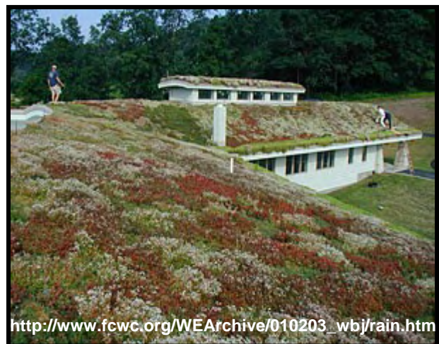
Figure 1: Green roof installed on a sloped roof
