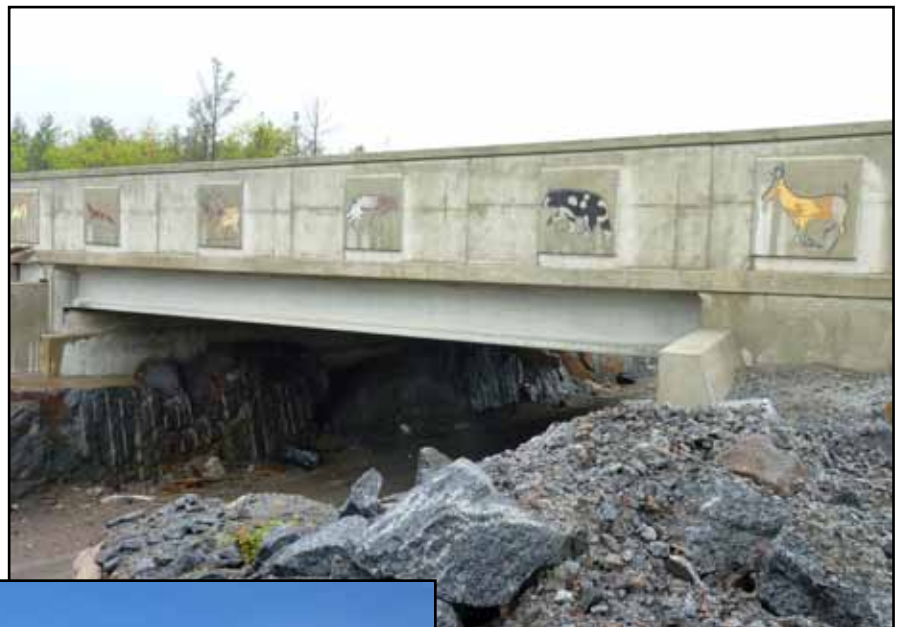
Wildlife crossing structures under construction in Ontario. The highway was realigned/twinned and this overpass (above) is the first of its kind in Canada east of the Rockies, 2011. The 5m X 5m underpass (left) is intended to be a joint wildlife/forest access structure. Photos by Ontario Ministry of Natural Resources.
