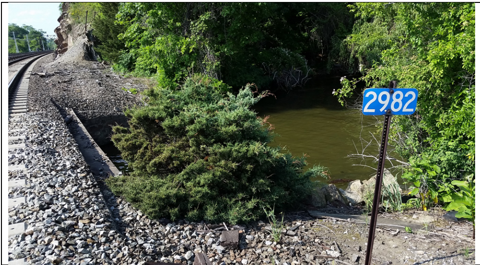
Figure 8: Sparta Brook MTA railroad underpass. Looking north
