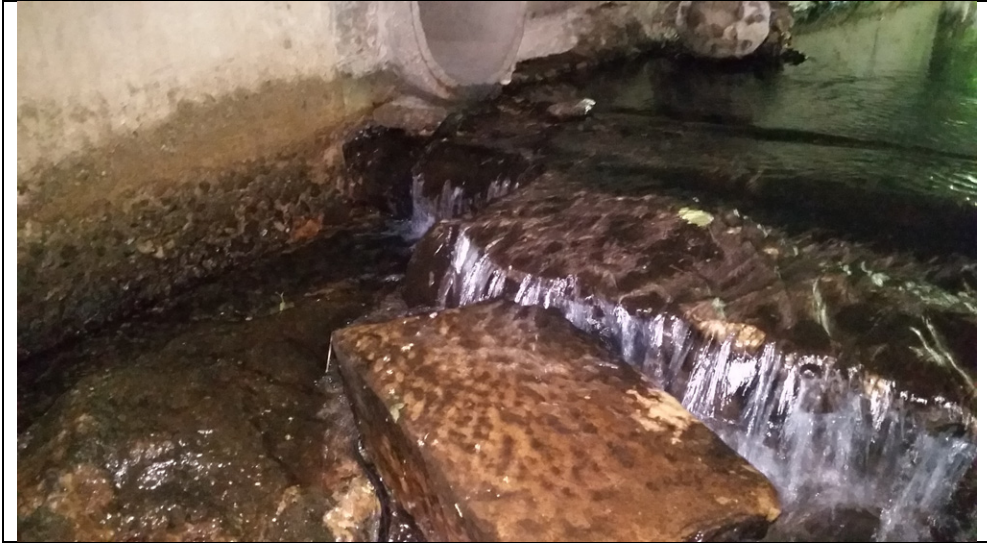
Figure 12: Sparta Brook. Second potential barrier to fish migration, left side. First real barrier.
