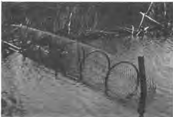
FIGURE 1. A PROPERLY INSTALLED BEAVER POND LEVELER
