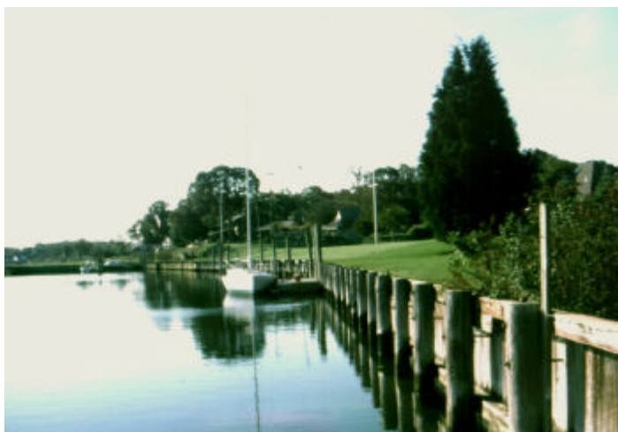
Figure 9. Bulkheaded shoreline of a tidal creek.
