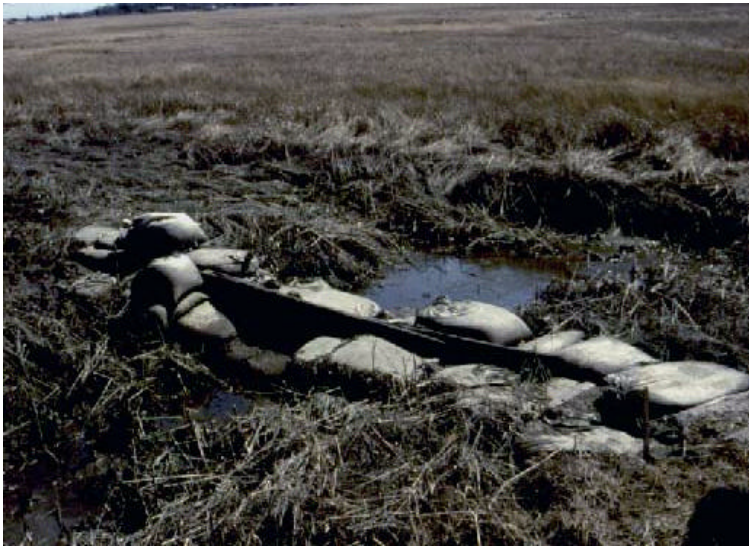
Figure 11. Ditch plug in an OMWM system.
