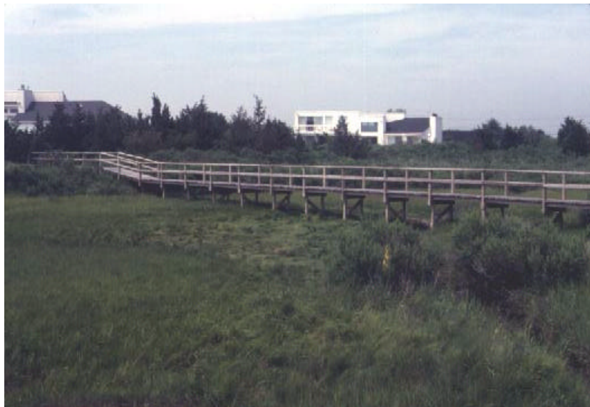
Figure 10. Walkway to a dock constructed over salt marsh.
