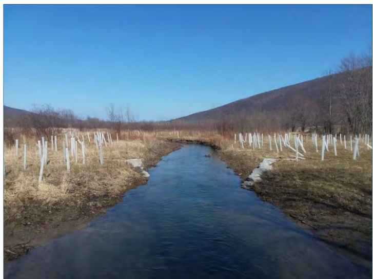
Photo 16: The Inlet restoration project excavated a new stream channel through old fields, and trees were planted to stabilize banks and establish a future riparian forest.
