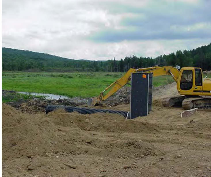
Photo 1. Water control structure being installed for wetland restoration project.
