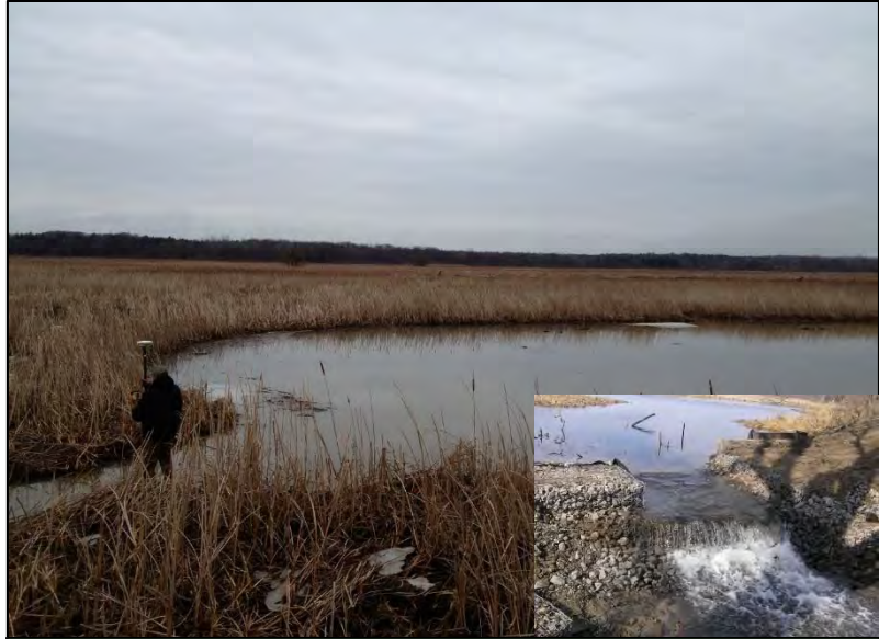
Manmade pothole and gabion rock water control structure at Lakeview WMA.
