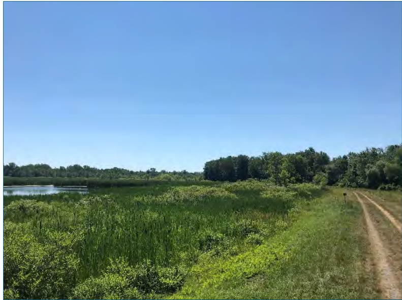
Photo 1: Earthen dikes divide wetland impoundments on the WMA and water control structures are used to manipulate water levels.
