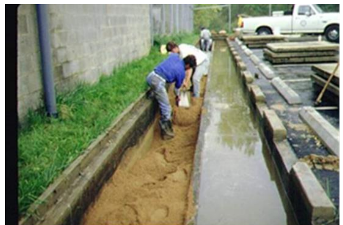
Figure 12.20 Example Concrete Perimeter Sand Filter (photo shows the filter with the grate top off as the filter is being maintained. Sedimentation chamber filled with water is on the right, and the sand filter chamber is on the left.)
