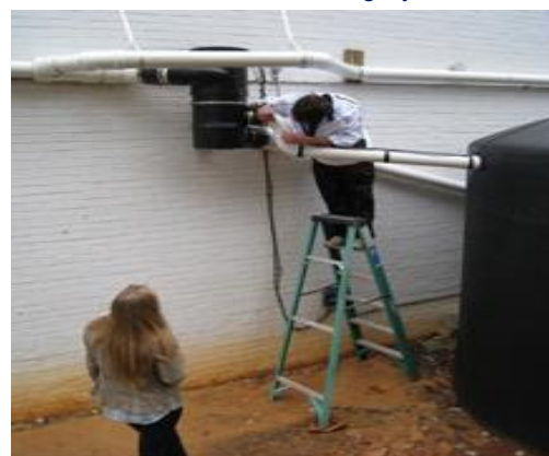
Figure 12.10 Inspecting the conveyance system, vortex-style filter.
