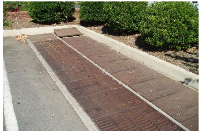
Figure 12.19 Example Perimeter Sand Filter
