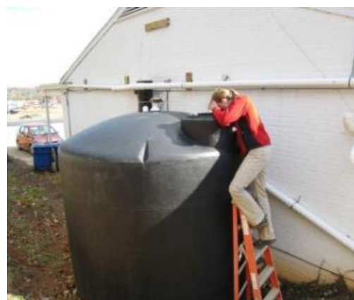
Figure 12.11 Inspecting the RWH system top access port.
