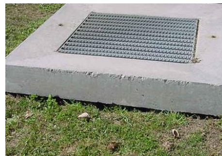
Water is “piping” down to the underdrain at the weak spot where the filter media meets the concrete overflow structure.
