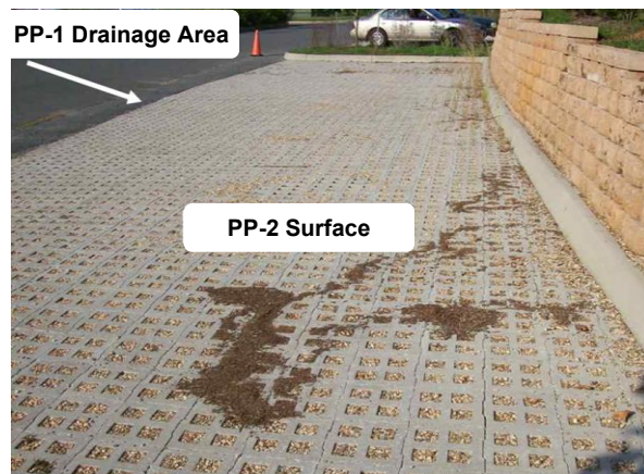
Figure 12.12 Key Areas for Level 1 Inspection of Porous Pavement
