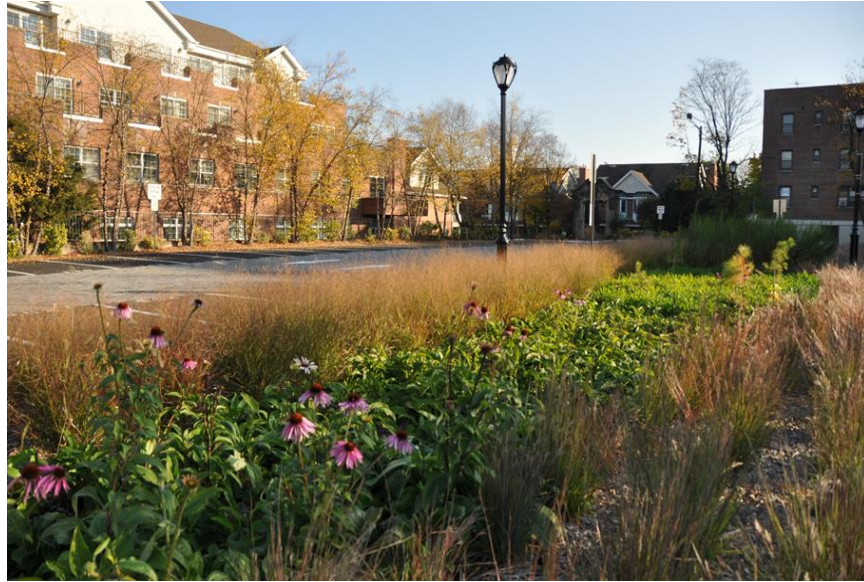
Figure 11.2 Parking Lot Bioretention (Photo Source: NYSEFC)
