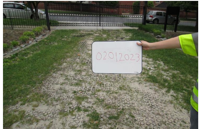
Figure 12.3 Use a white board and digital camera to note SMP tracking #, date of inspection, and other forms of documentation. Alternatively, tag photographs using a smartphone
