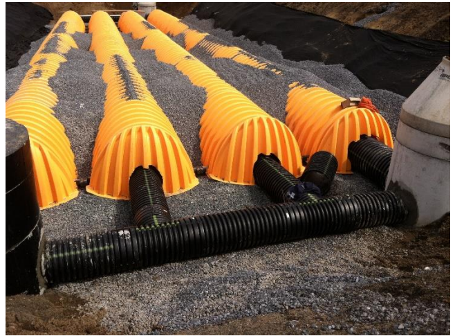
Figure 8.17 Underground infiltration system installed in Mahopac, NY
