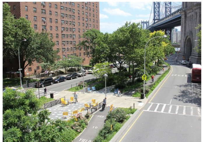
Figure 8.7 Rain Gardens installed in Manhattan, NY
