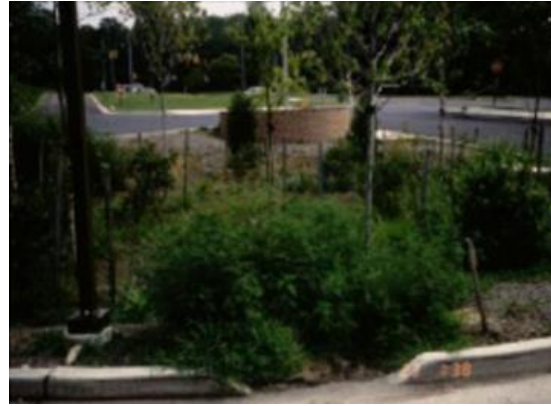
Curb Inlet #2: flow enters through drop curb.
