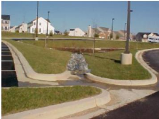
Curb Inlet #1: flow enters through curb channel.
