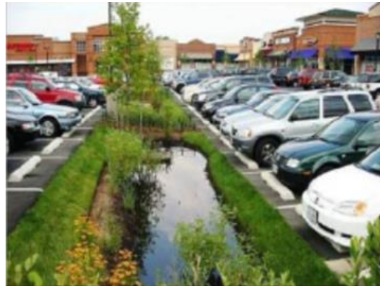
Grass filter strip: sheet flow enters and is evenly distributed along the practice length.
