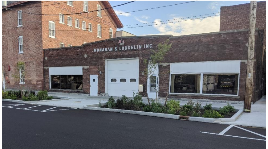
Figure 8.4 Tree Trench installed in Hudson Falls, NY
