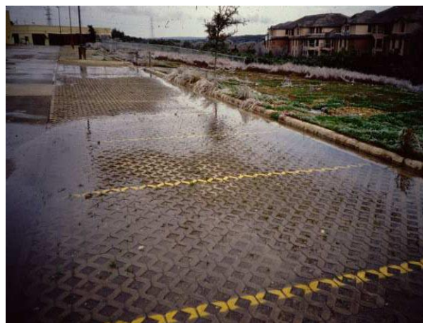
Figure 12.13 Winter salting, sanding, plowing, and snow storage can cause problems for porous pavement surfaces, which may trigger a Level 3 Inspection.
