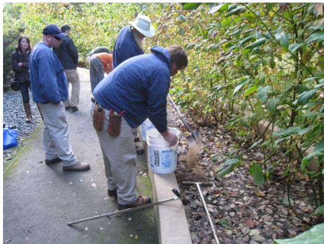
Adding sand to a wick drain. The vertical perforated PVC pipe has already been placed in the auger hole.
