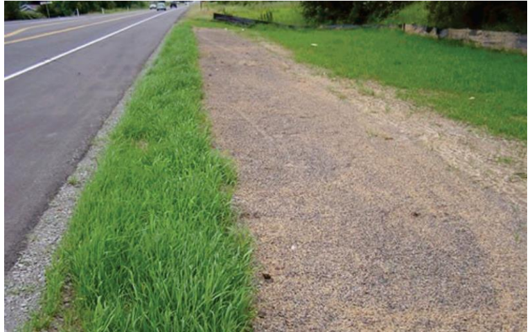
Figure 8.16 Bioslope Application (Georgia Stormwater Management Manual, 2016 Edition)
