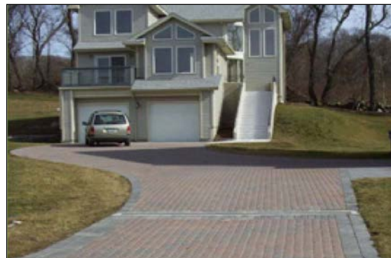
Figure 5.21 Permeable pavers as an alternative driveway surface
