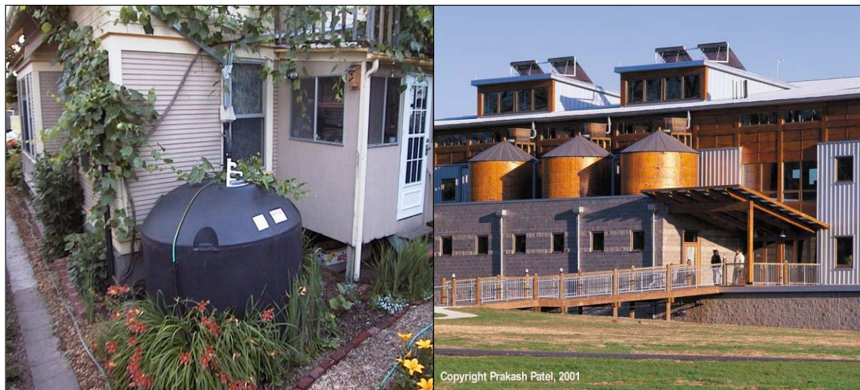
Figure 5.55 Cisterns can be designed for smaller residential uses (left) or for larger commercial and industrial business operations (right).
