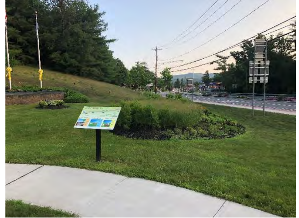
Figure 8.6 Rain Garden installed in Lake George, NY
