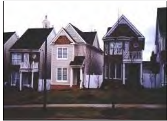
Figure 5.28 Taller houses create a smaller impervious footprint (Source: Center for Watershed Protection, 2005)
