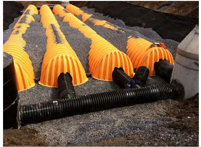
Figure 8.17 Underground infiltration system installed in Mahopac, NY
