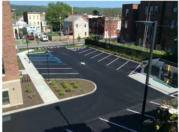
Figure 8.9 Porous Asphalt parking stalls installed in Cohoes, NY
