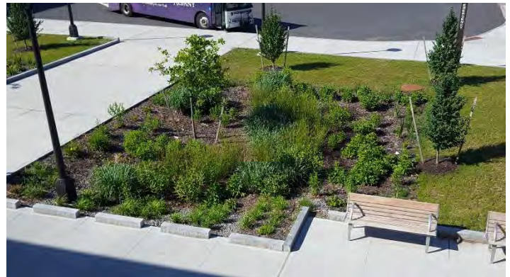
Figure 8.7 Rain Gardens installed at SUNY Albany campus
