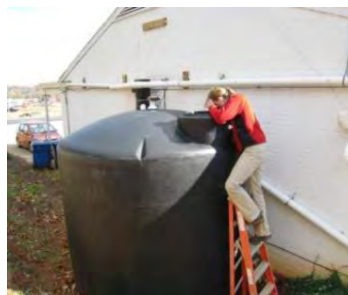
Figure 12.11 Inspecting the RWH system top access port.
