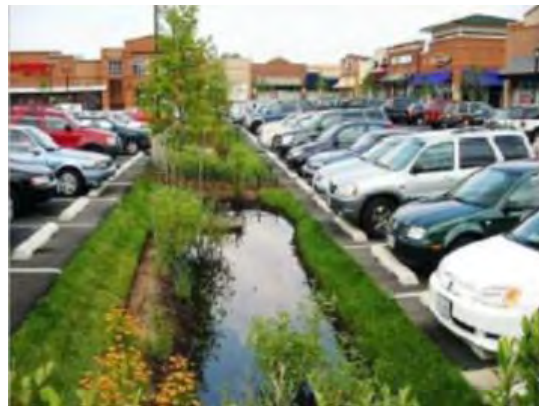
Grass filter strip: sheet flow enters and is evenly distributed along the practice length.
