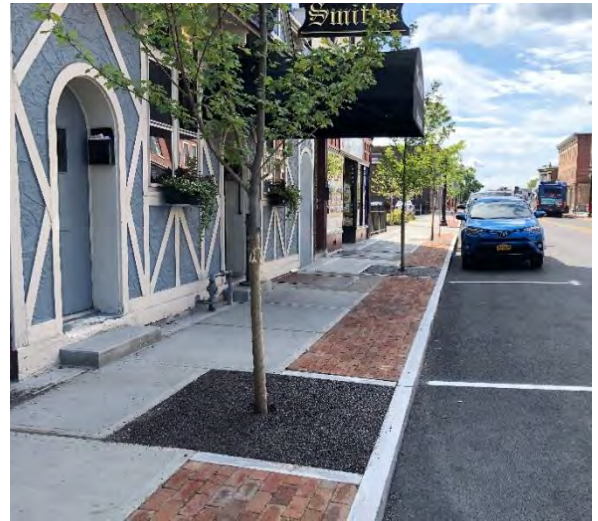
Figure 8.2 Tree Pit installed in Cohoes, NY
