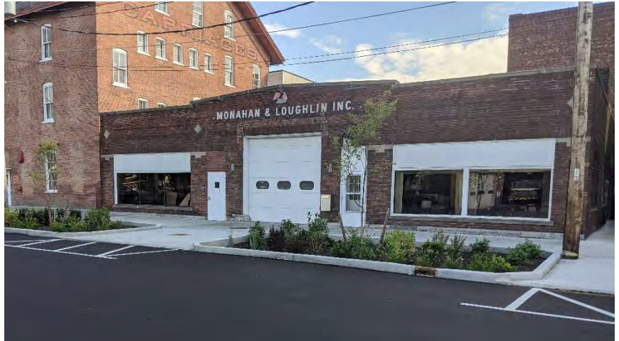
Figure 8.4 Tree Trench installed in Hudson Falls, NY
