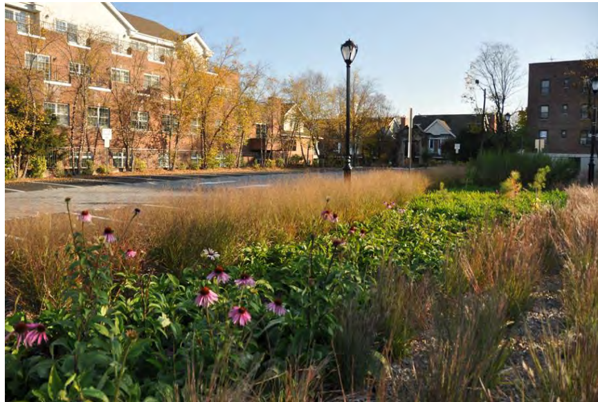
Figure 11.2 Parking Lot Bioretention (Photo Source: NYSEFC)
