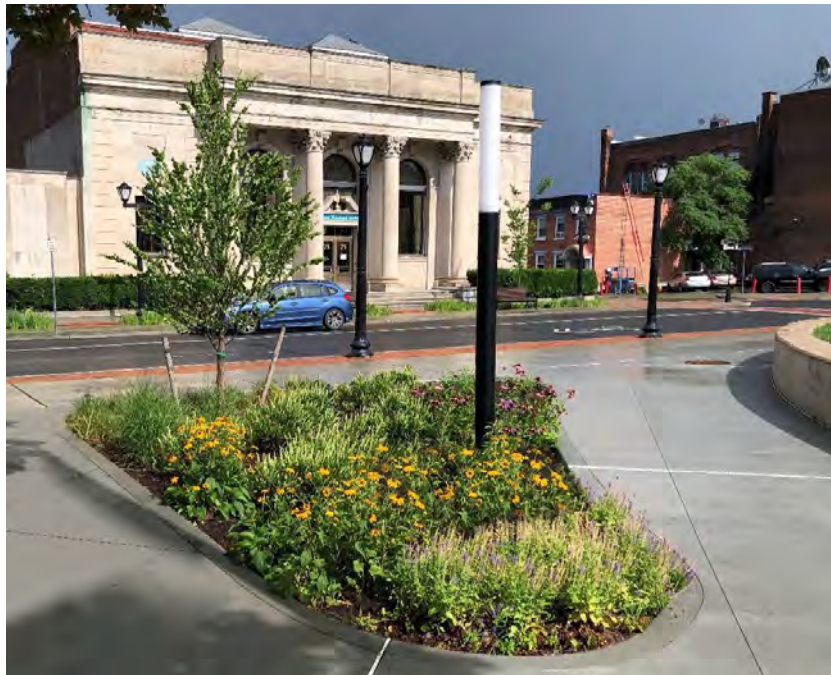
Figure 11.6 Canal Square Park Rain Garden (Photo Source: City of Cohoes/NYSEFC)
