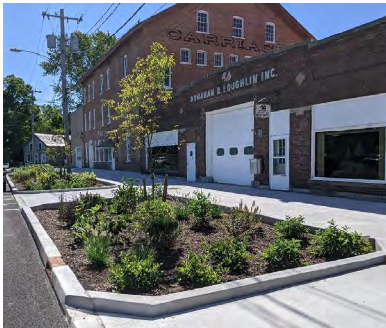
Figure 11.5 Locust Street/ Paris Park Tree Trench (Photo Source: Village of Hudson Falls/NYSEFC)
