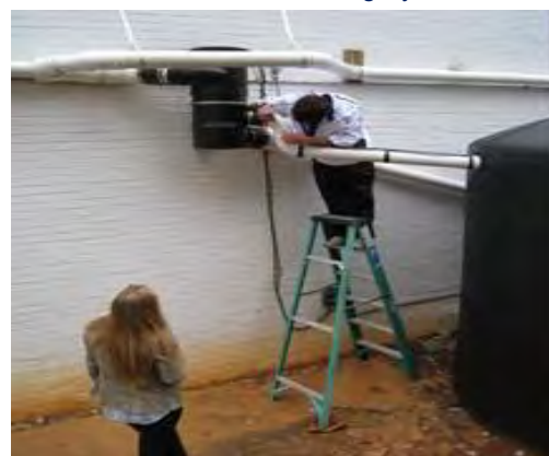
Figure 12.10 Inspecting the conveyance system, vortex-style filter.
