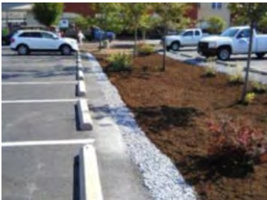
Pea Gravel Diaphragm: sheet flow enters and is evenly distributed along the practice length.
