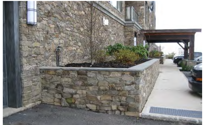
Figure 8.8 Stormwater Planter installed in Tarrytown, NY
