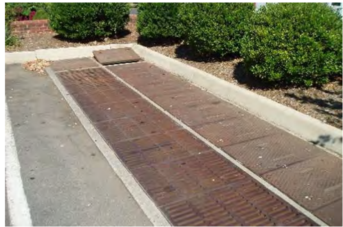
Figure 12.19 Example Perimeter Sand Filter
