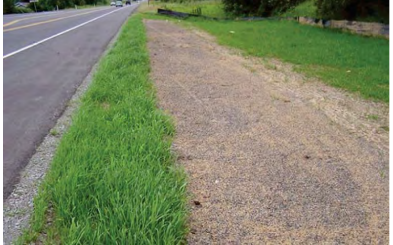
Figure 8.16 Bioslope Application (Georgia Stormwater Management Manual, 2016 Edition)
