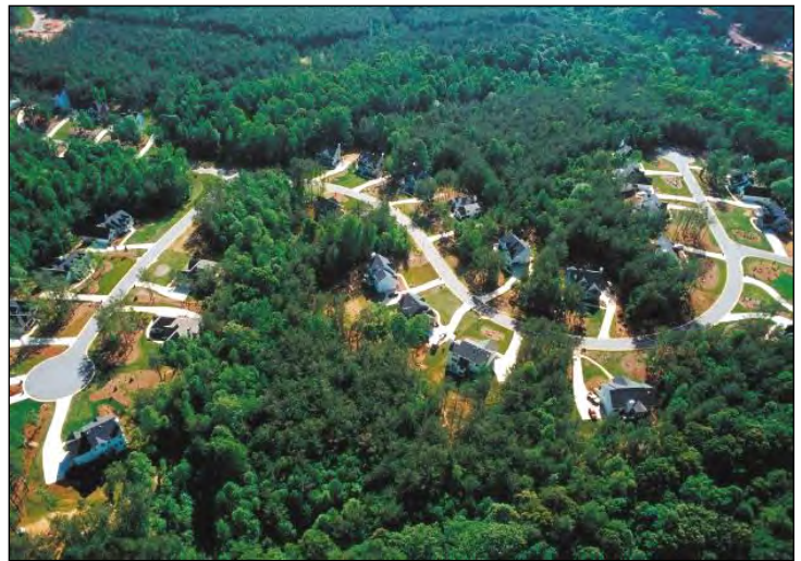
Figure 5.11 Aerial view of an open space or “cluster” subdivision (Source: Georgia Stormwater Manual, 2001)
