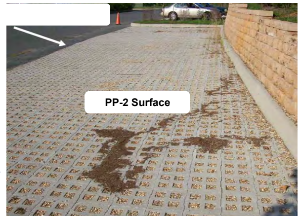
Figure 12.12 Key Areas for Level 1 Inspection of Porous Pavement
