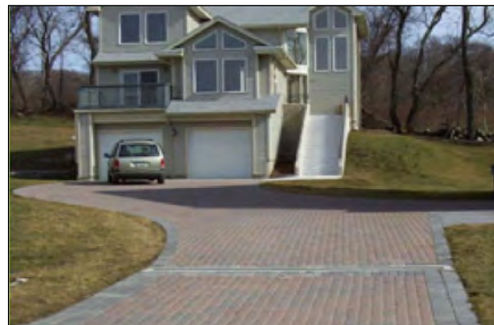
Figure 5.21 Permeable pavers as an alternative driveway surface
