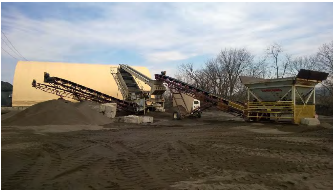
Figure 8. Fines Processing Area
