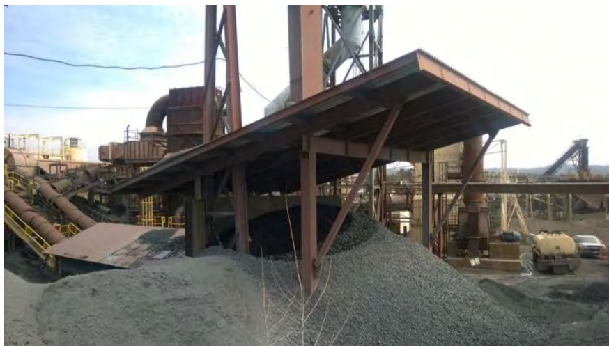
Figure 4. New Kiln Feed Storage Pile Enclosure
