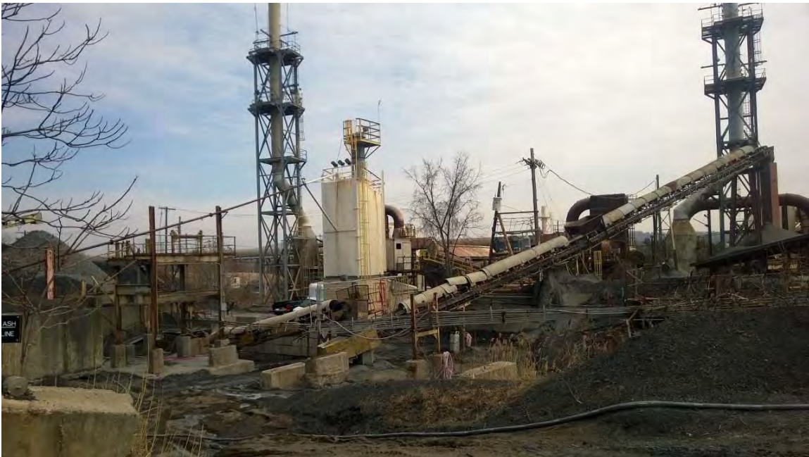
Figure 3. #4 and #5 Conveyors in the Kiln Feed Area
