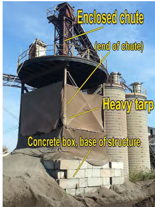
Photo 2. The enclosed fines structure, including chute coming in from above structure, tarp surrounding structure, and other structure details.
