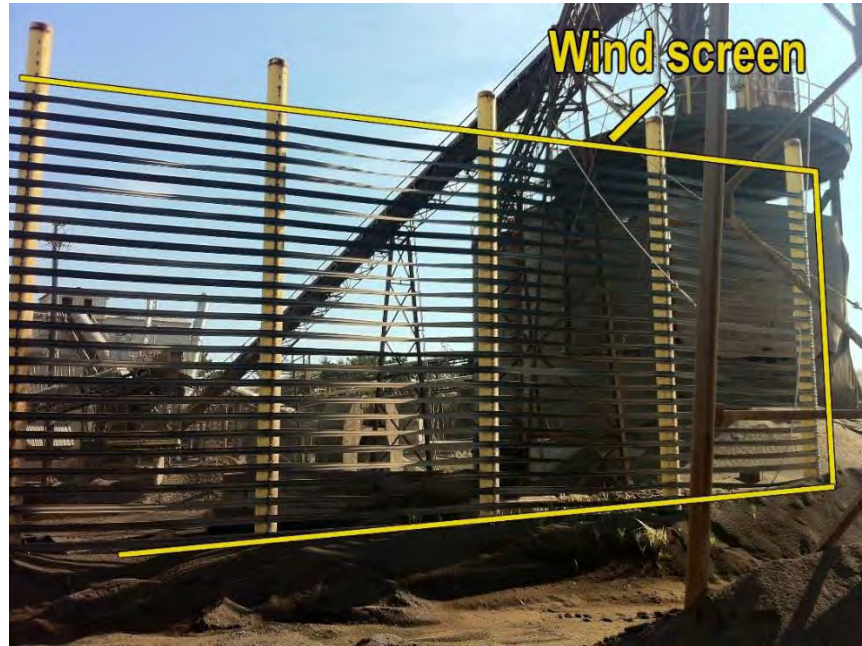
Photo 3. View of open fines area from western side, showing the wind screen.
