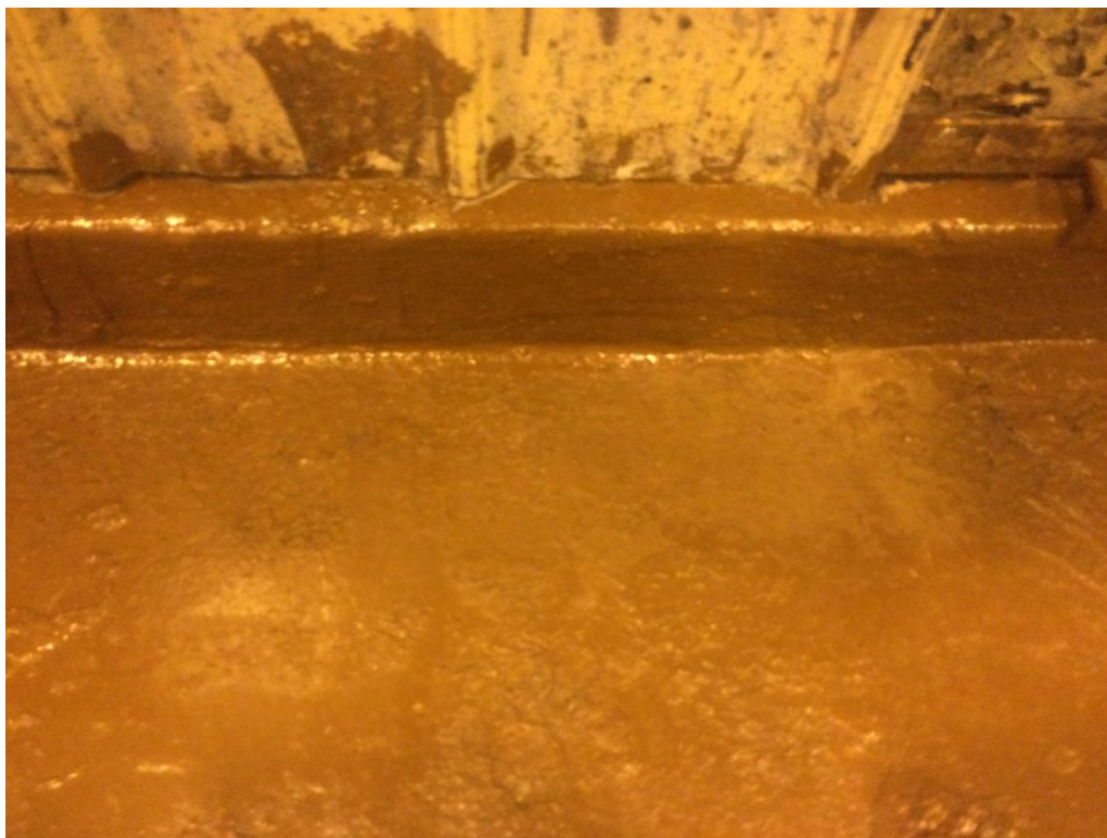
Close-up of Curb Repair along Interior Wall
