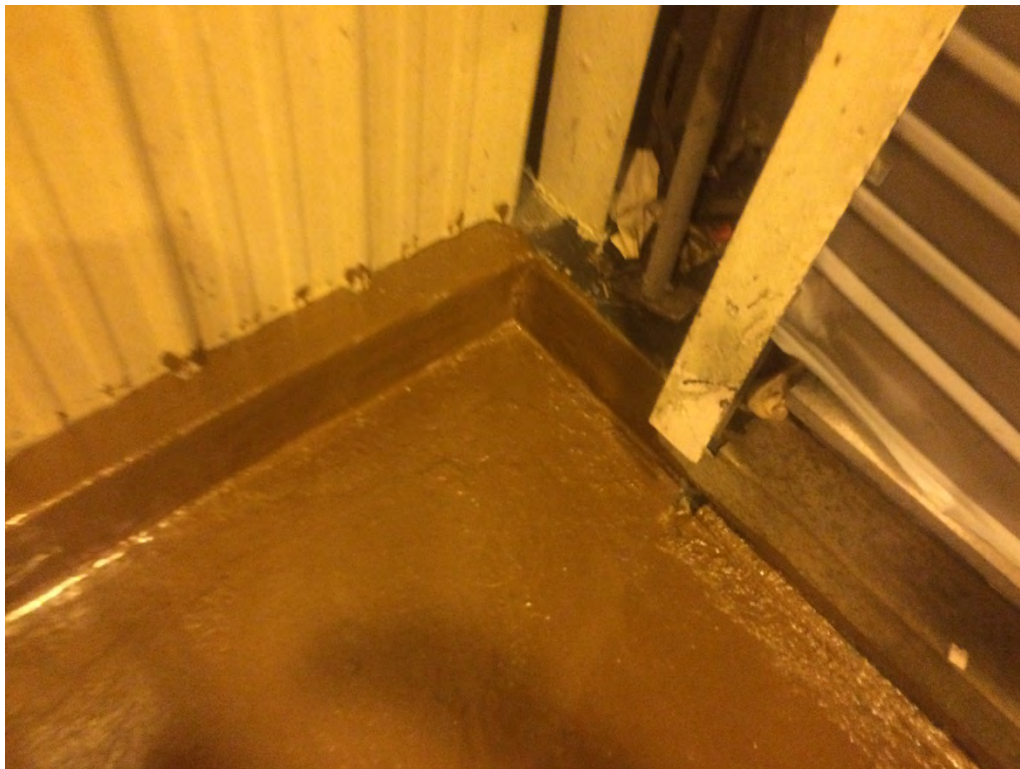
Close-up of Curb & Corner Repair at North Side Overhead Door
