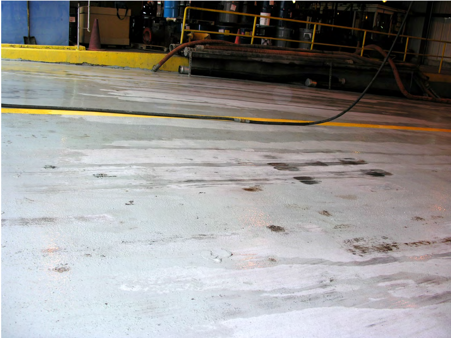
Unloading Area #2 of Materials Management Building Looking Northeast
