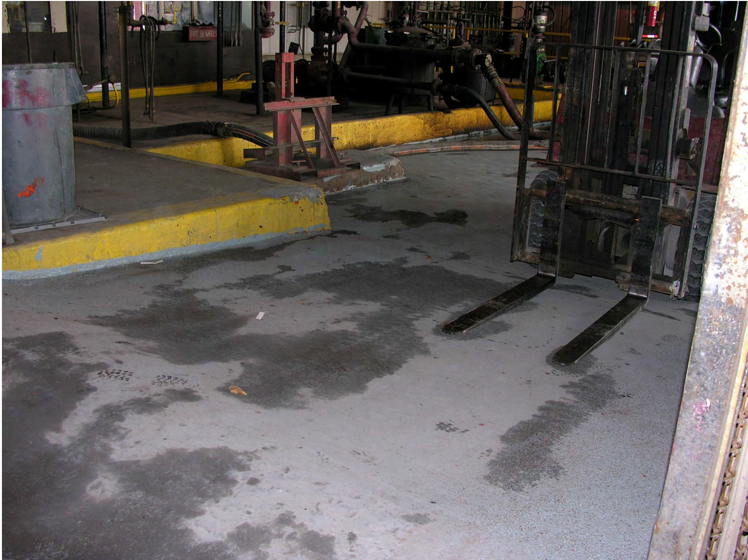
Drum Processing Building Access Ramp from Unloading Area #1
