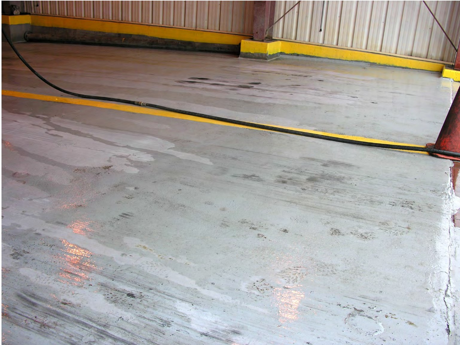
Western End of Unloading Area #2 Looking Southeast
