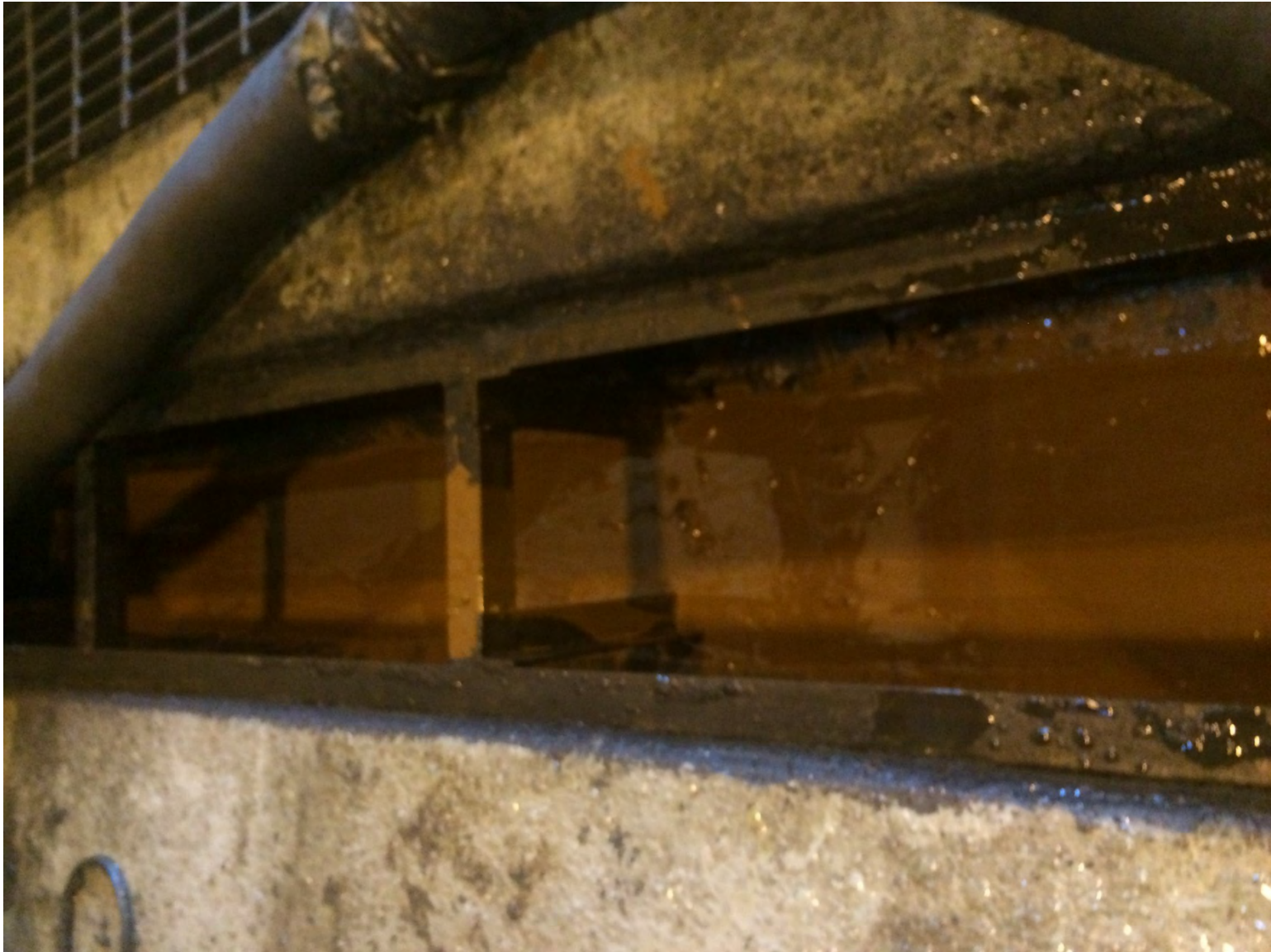
Unloading Area #2 Sump Trench
