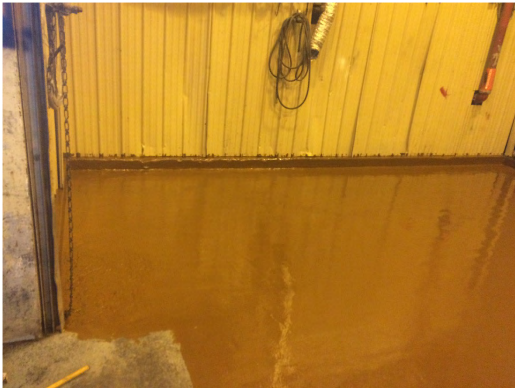
Southwest Corner of Drum Processing Building @ Entrance
