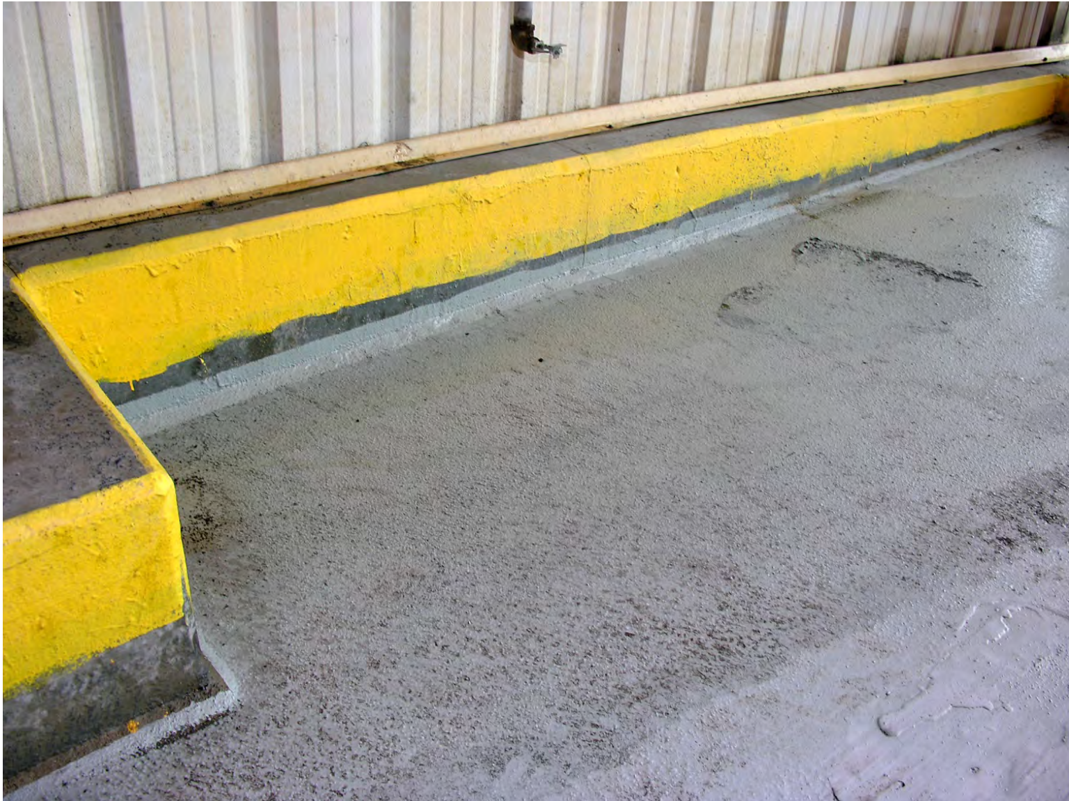
Southwest Curbing Showing Maintenance Coating and Floor Repairs
