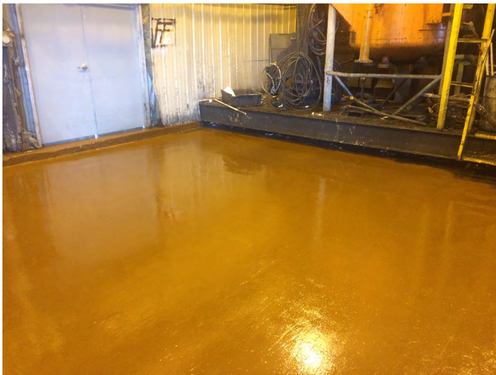
Drum Processing Building Looking Northeast from Unloading Area 1 Entrance
