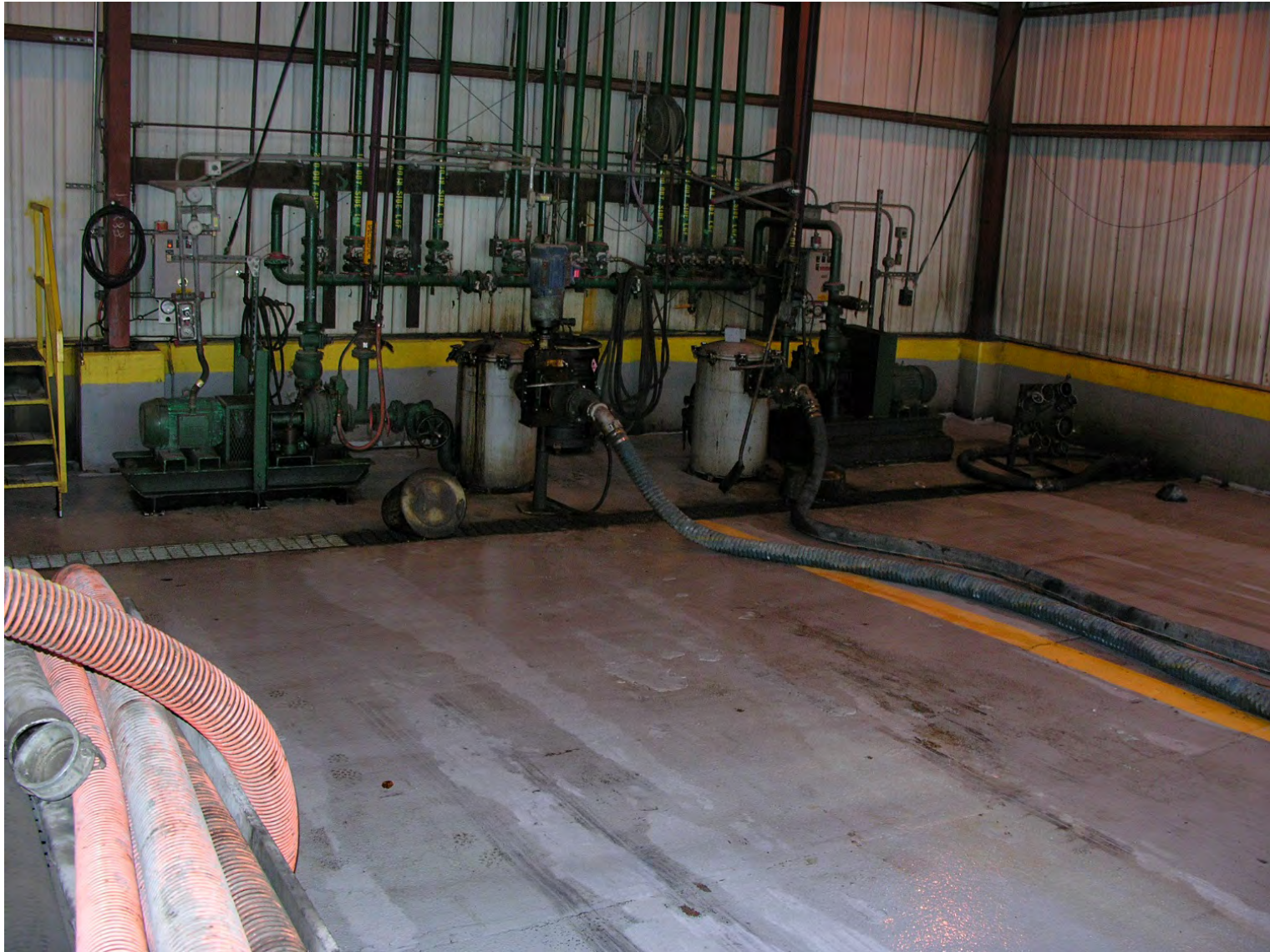
Unloading Area #2 Equipment End East
