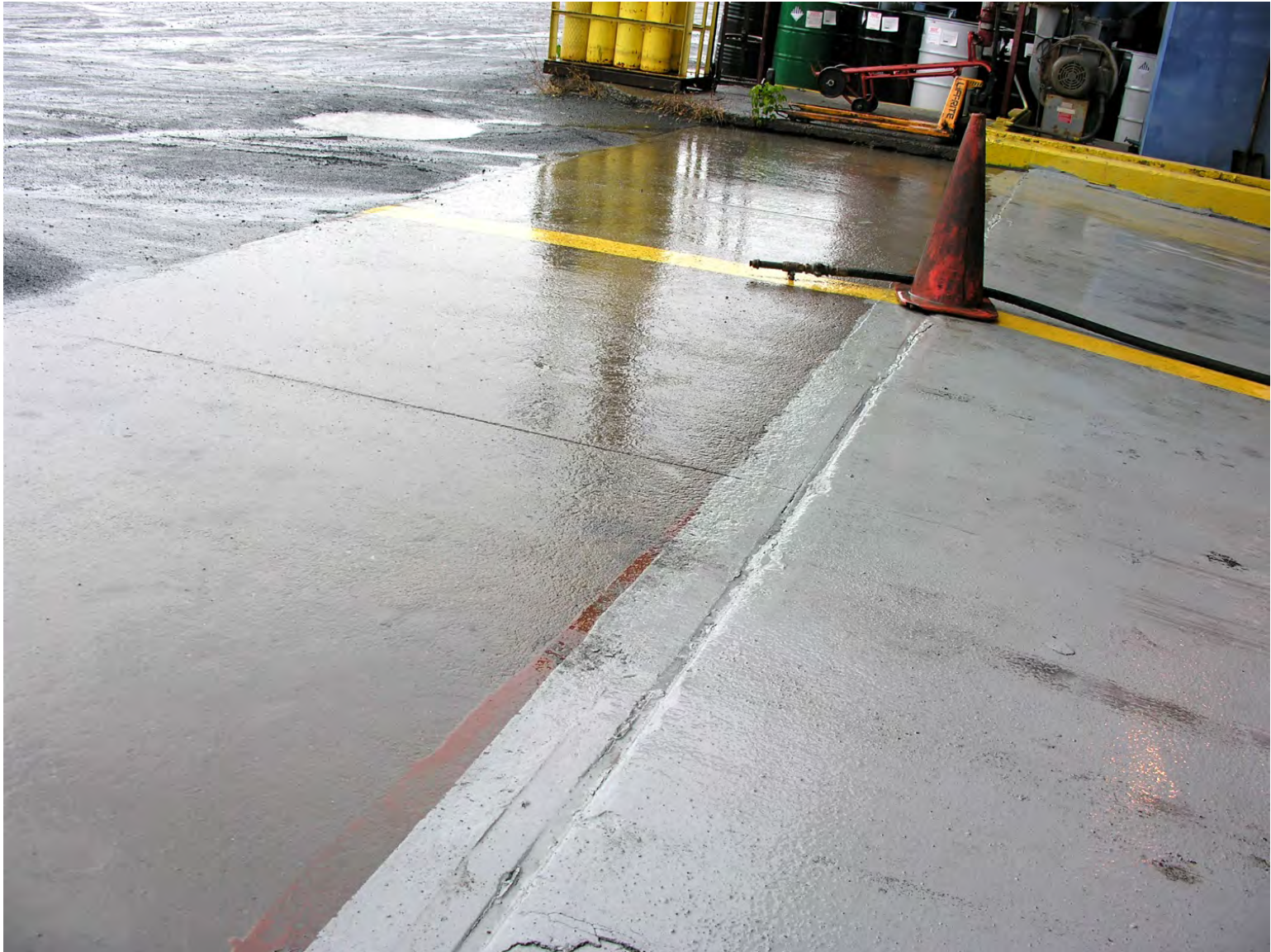
Entrance End of Unloading Area #2
