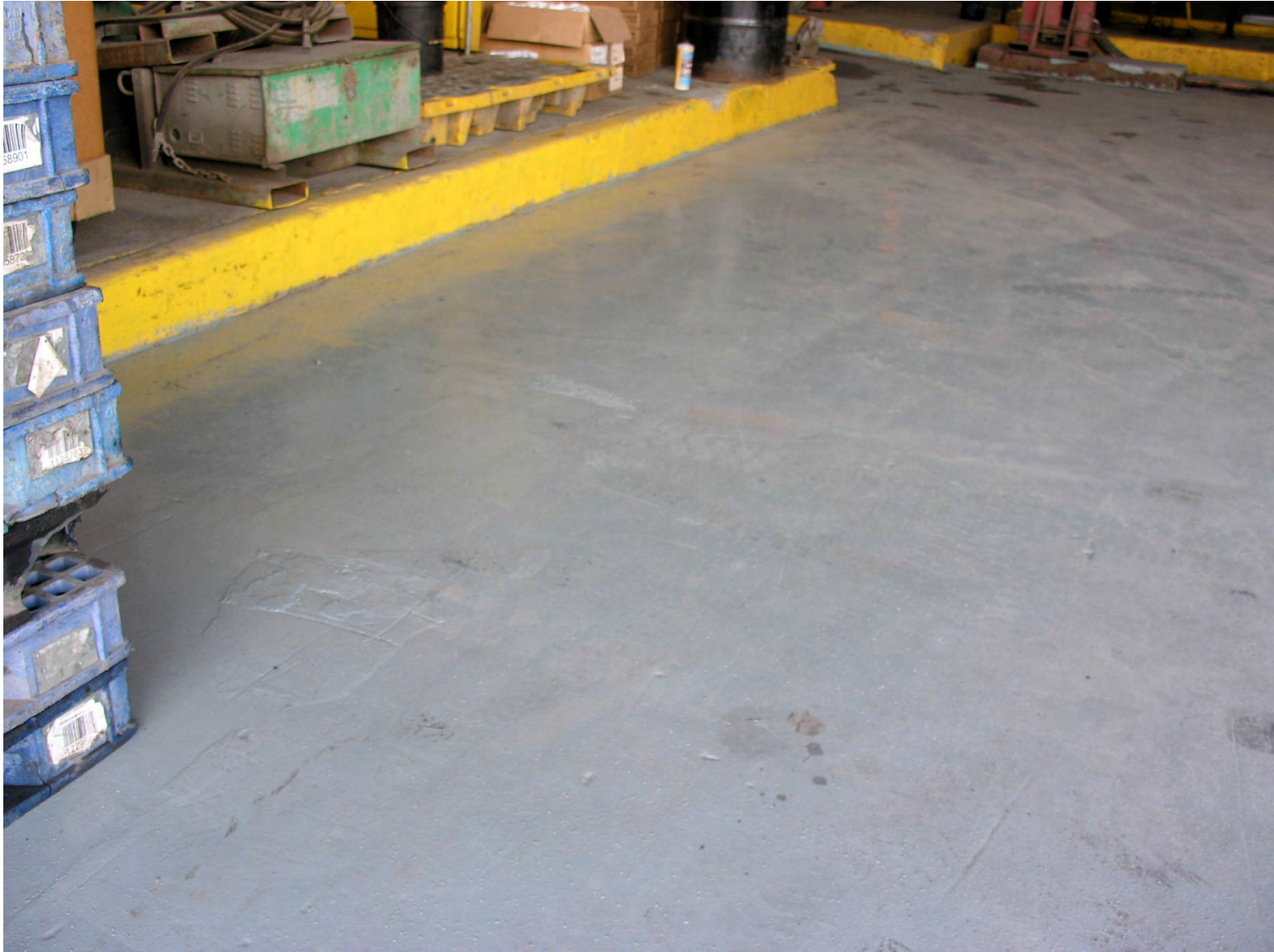
Unloading Area #1 North Side Looking Northeast
