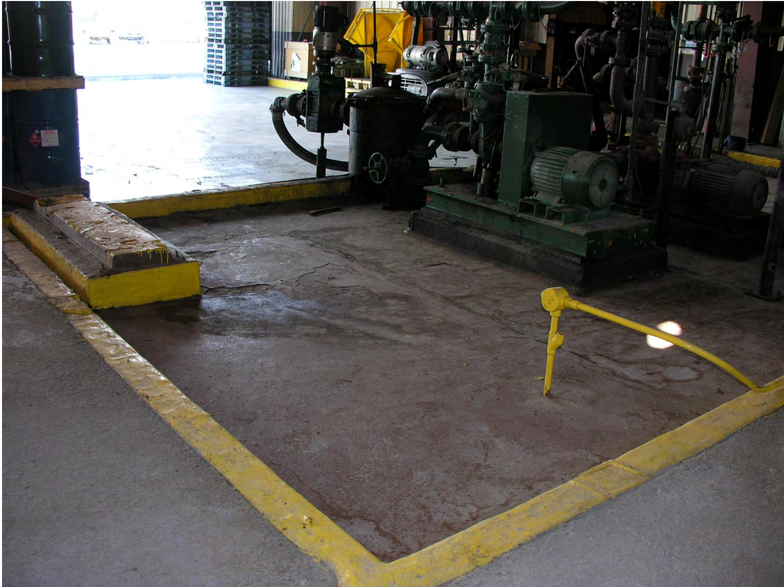
Unloading Area #1 Pumping Equipment Containment
