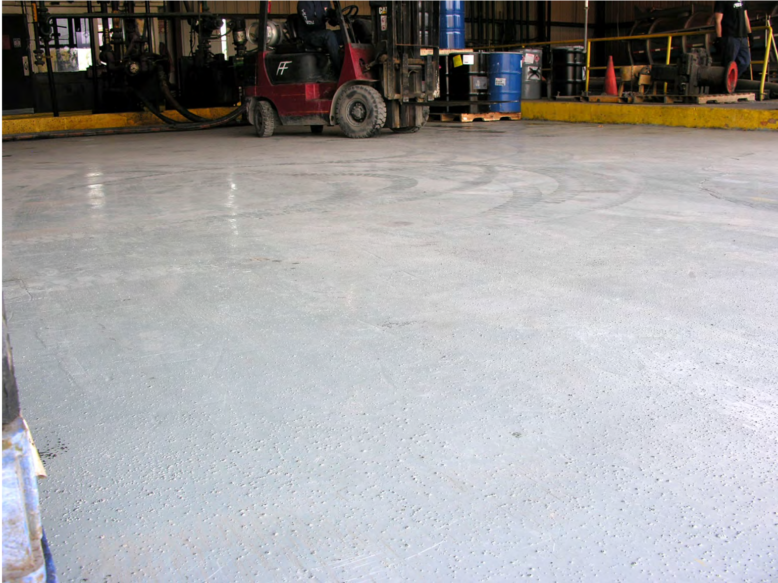
Unloading Area #1 (North) with Most Recent Maintenance Coating
