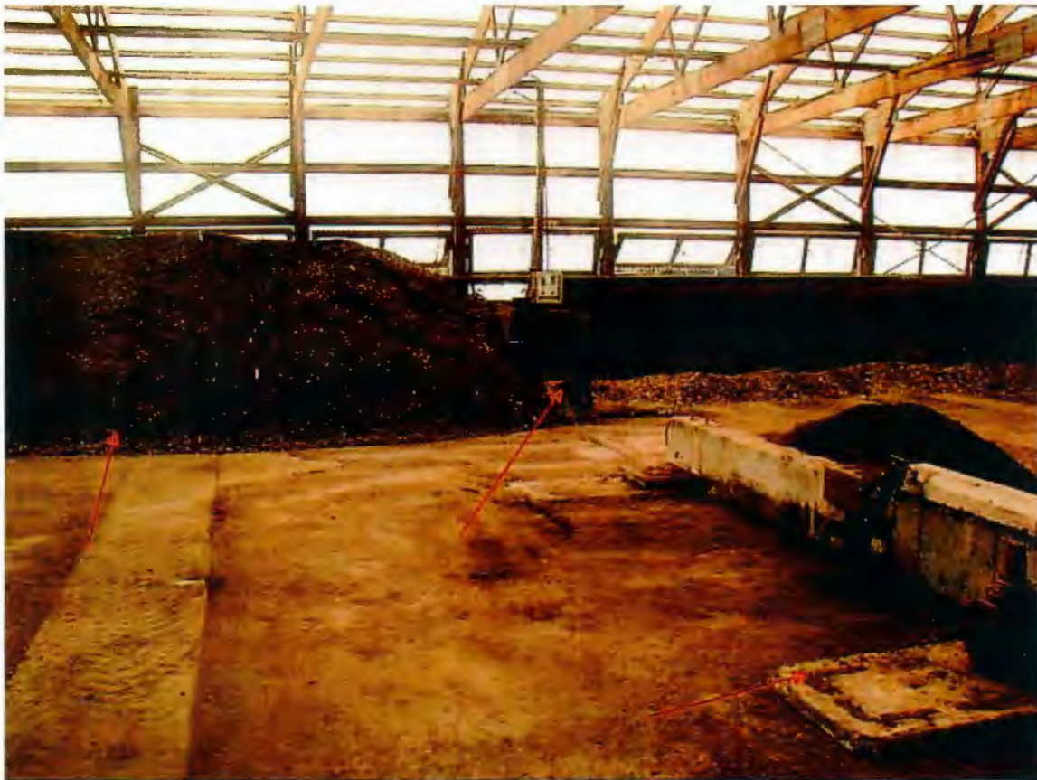
Active pile on left. New pile to be created on right
