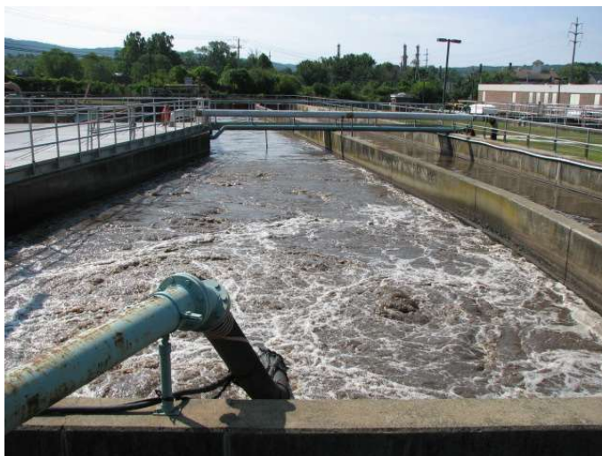
Figure 6: Oxidation Ditch
