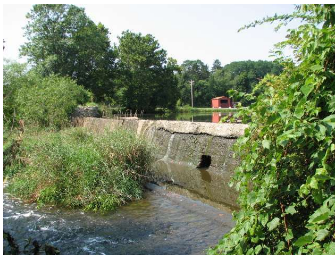
Figure 5: View from Outfall 001
