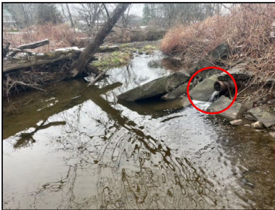
Outfall Location and Image
