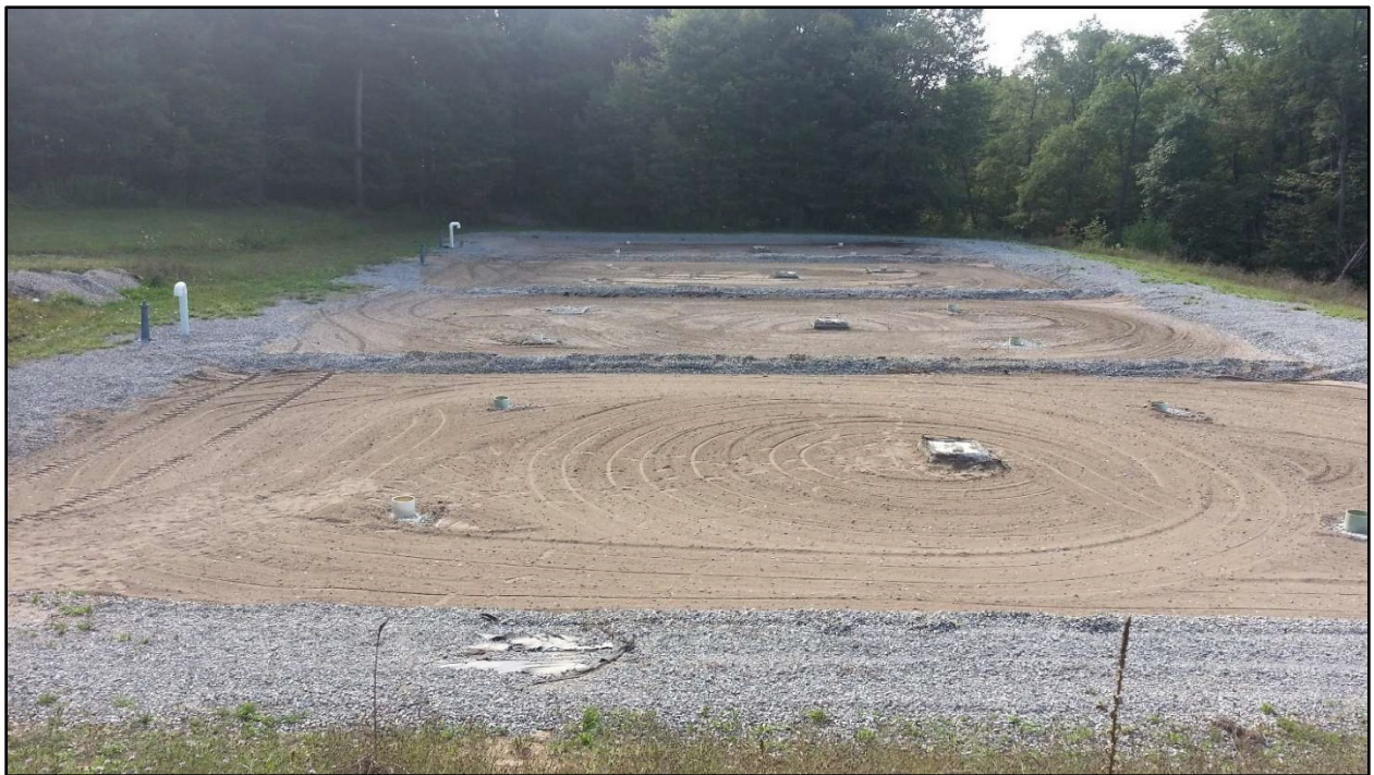
Figure 3. Forestport WWTP Sand Filter Beds
