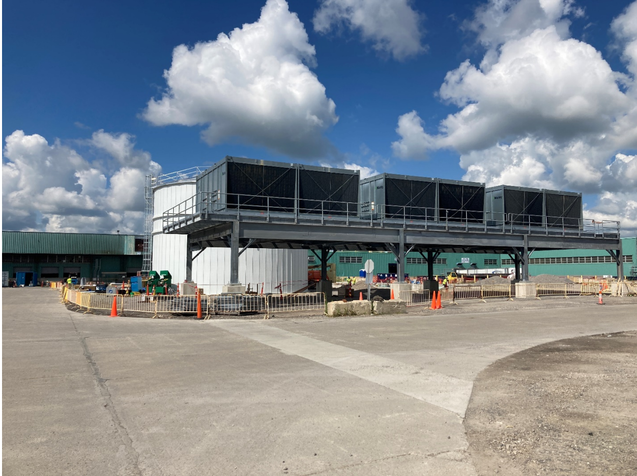
Figure 4: Elevated Cooling Tower Structure
