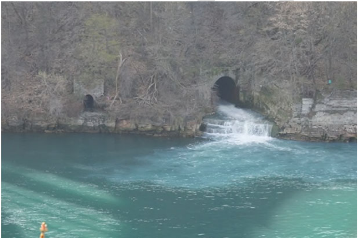
Figure 4: Outfall 001 (right); Falls Street Tunnel CSO Outfall 003 (left).
