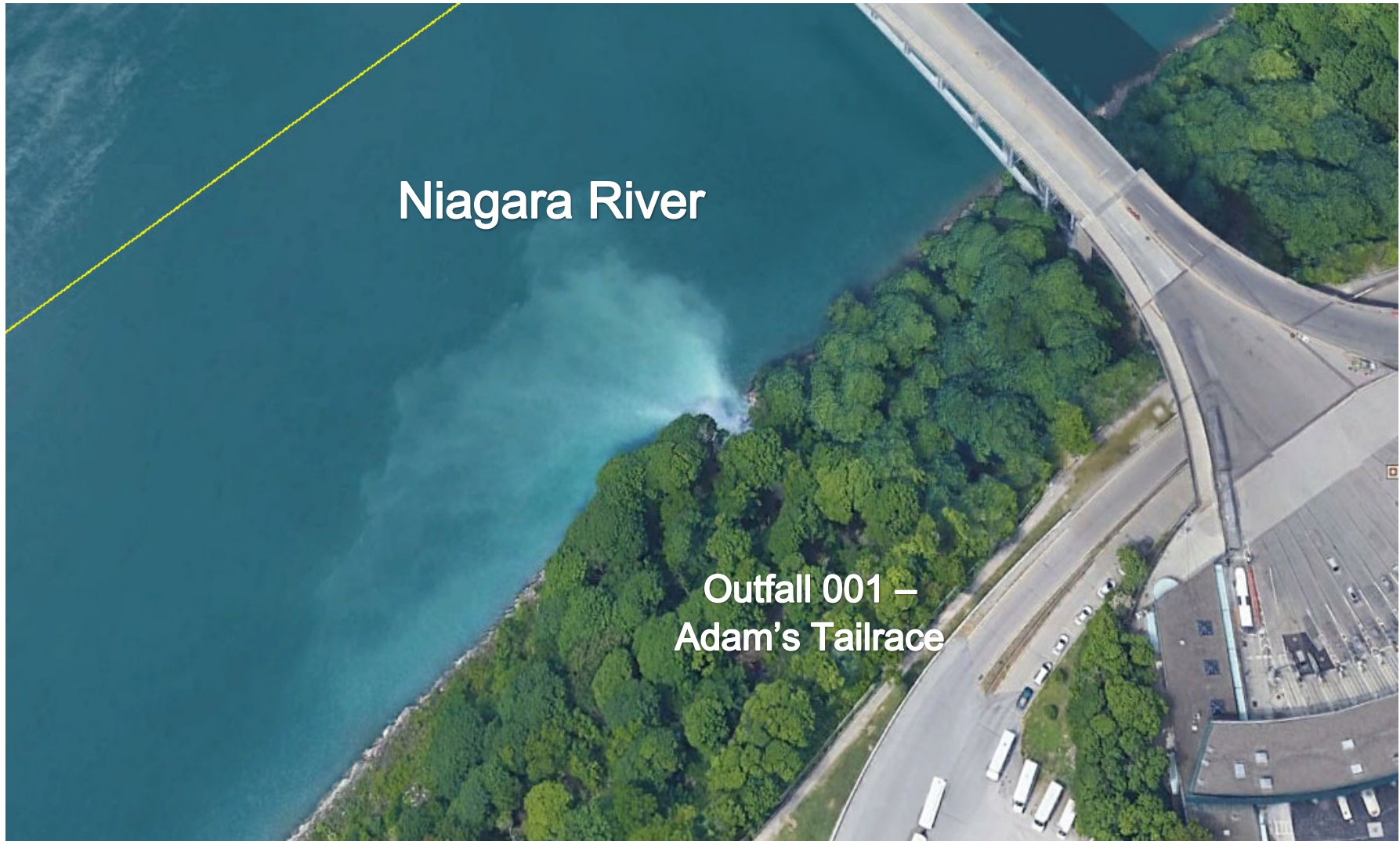
Figure 3: Aerial view of Outfall 001 to the Niagara River.
