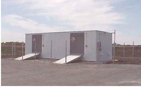
Figure 7-2. Hazardous Materials Storage Locker
