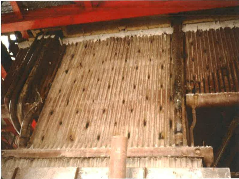
**Figure 1: Waterwall Furnace Section**
