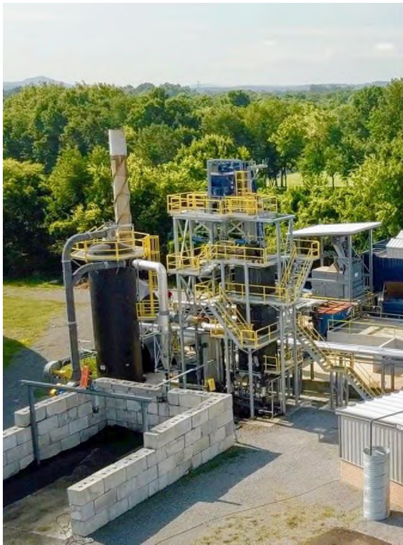
Gasification Plant in Lebanon, Tennessee (64 tpd, 1.8M kWh)
