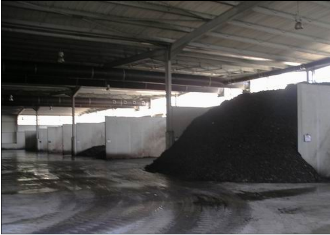
Photos 25 & 26 - Curing Bunkers in Shed
