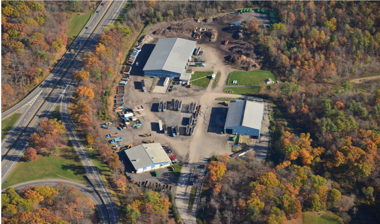
Ulster Transfer Station
